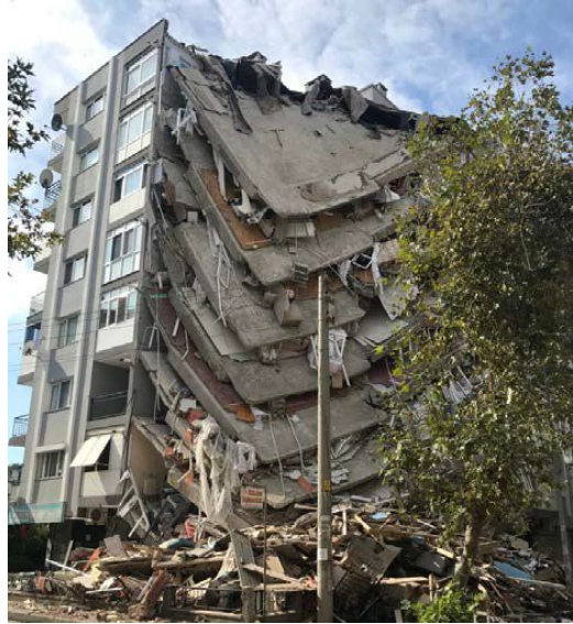
Partial collapse, pancake type, 8 story building 3
