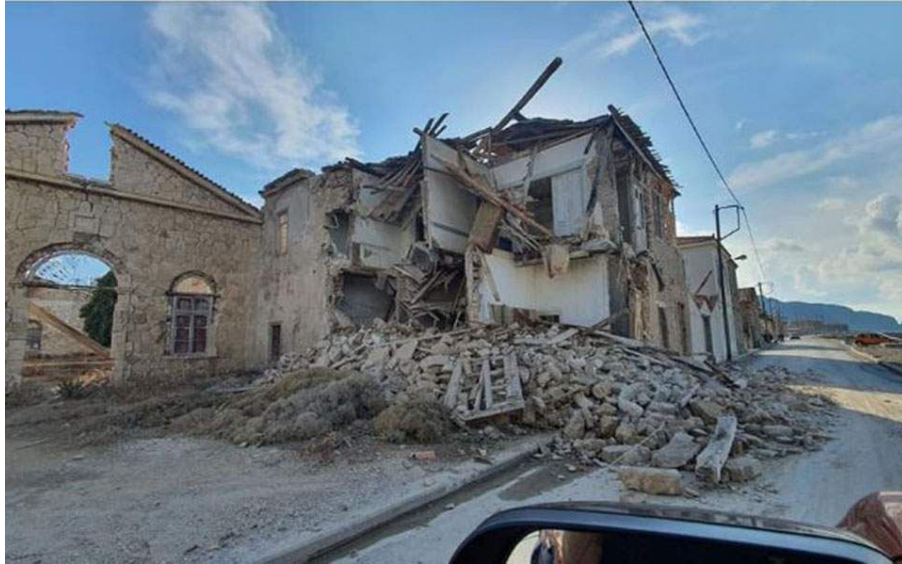
Collapsed old building in Samos (Greece) 9
