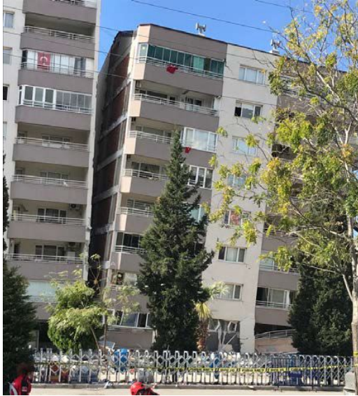
Failure of lower stories, ten story building 3
