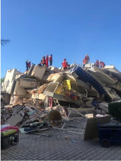
Pancake type collapse 7
