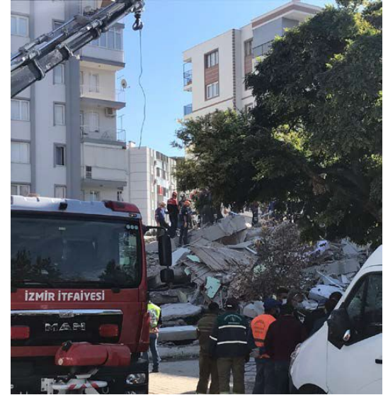
Collapsed eight story building 3
