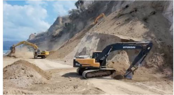
Excavator clears landslide on the Trans-Flores road (spanning Labuan Bajo–Ende–Mauwere) [8]
