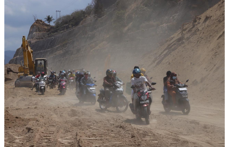
Trans-Flores Ende–Bajawa after landslide clearance, Aug. 20 [2]
