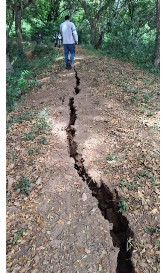
Levee cracks due to liquefaction Bolivar, Cauca Valley
