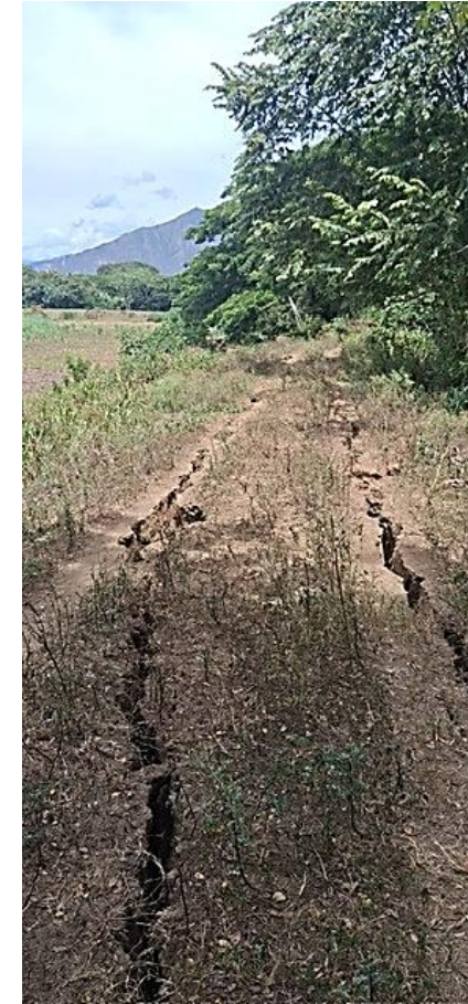
Levee cracks due to liquefaction Bolivar, Cauca Valley
