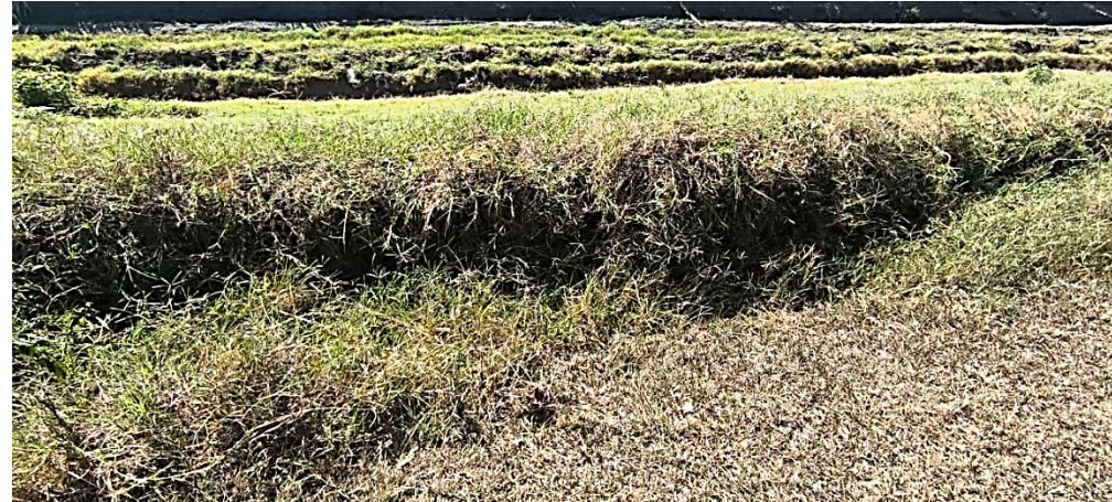
Levee cracks due to liquefaction at corregimiento El Overo, Bugalagrande, Cauca Valley
