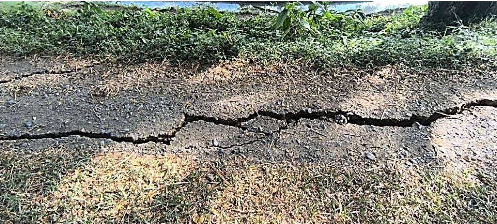
Levee cracks due to liquefaction at corregimiento El Overo, Bugalagrande, Cauca Valley
