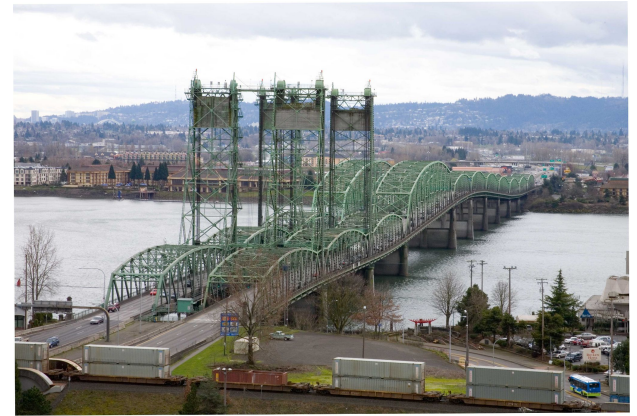
Columbia River I-5 Bridge
