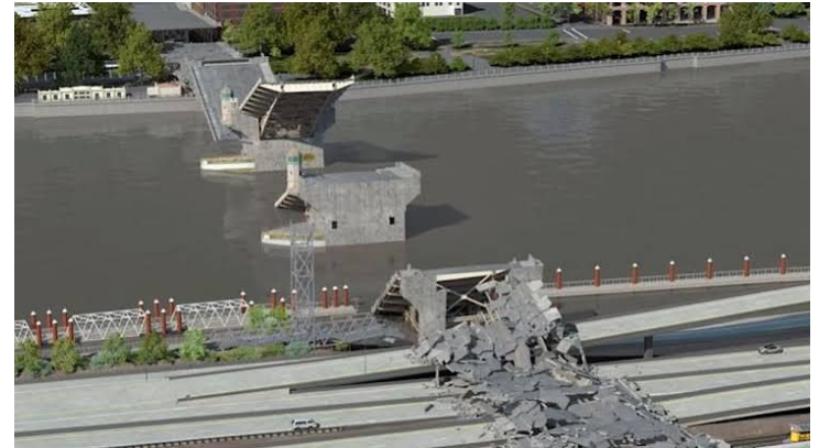
Collapse of Burnside Bridge in EQ (simulated by Multnomah County)
