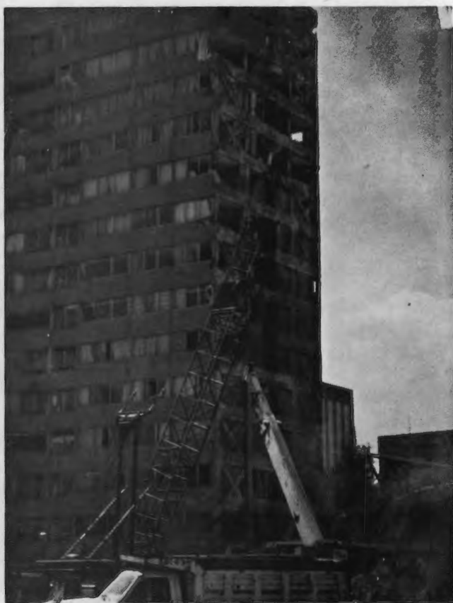
Nuevo Leon Housing Project showing the braced wall adjoining the building completely collapsed.
