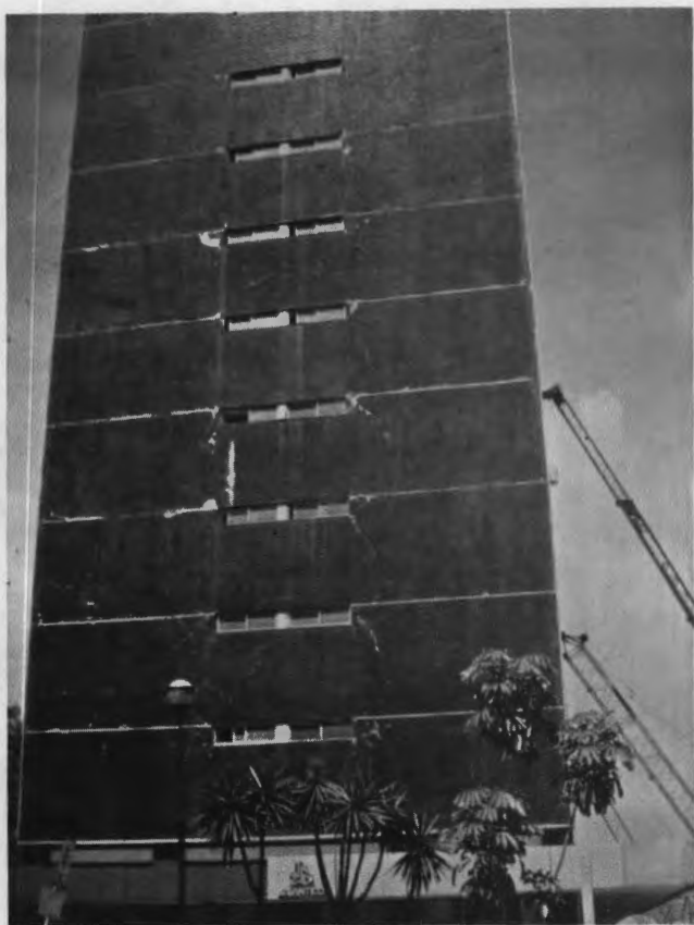
Nuevo Leon Housing Project -- remaining building end wall showing open first floor. The back of this building collapsed completely and caused many deaths.
