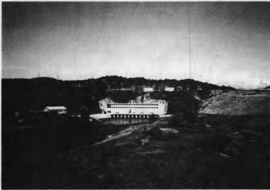
photo: EQE, Inc.
