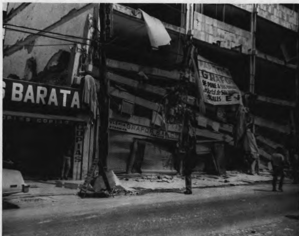
7-story commercial building -- lower floor collapse
