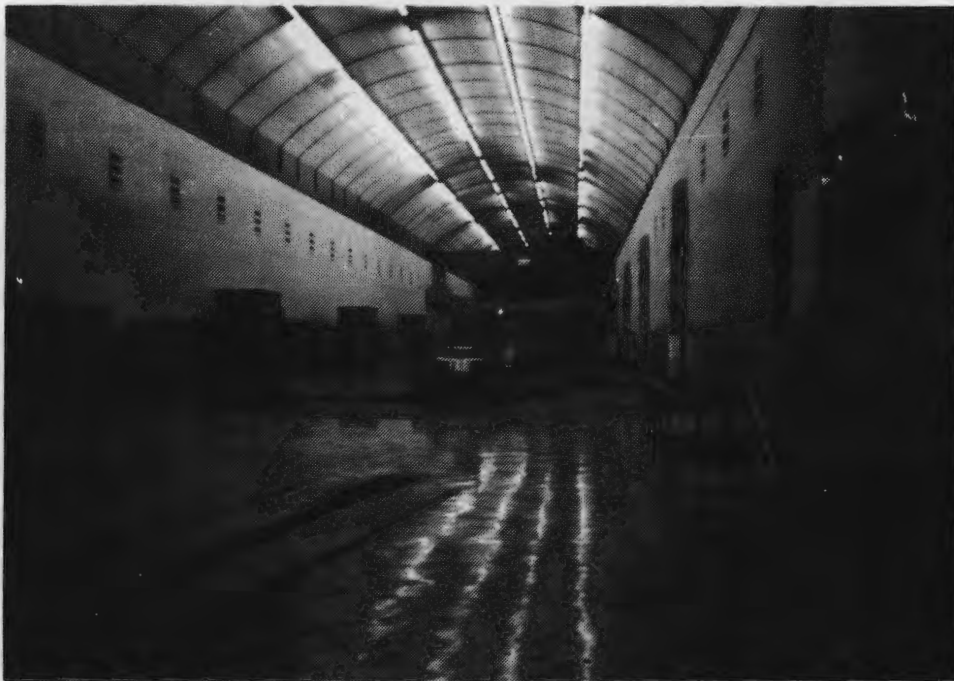
photo: EQE, Inc.
