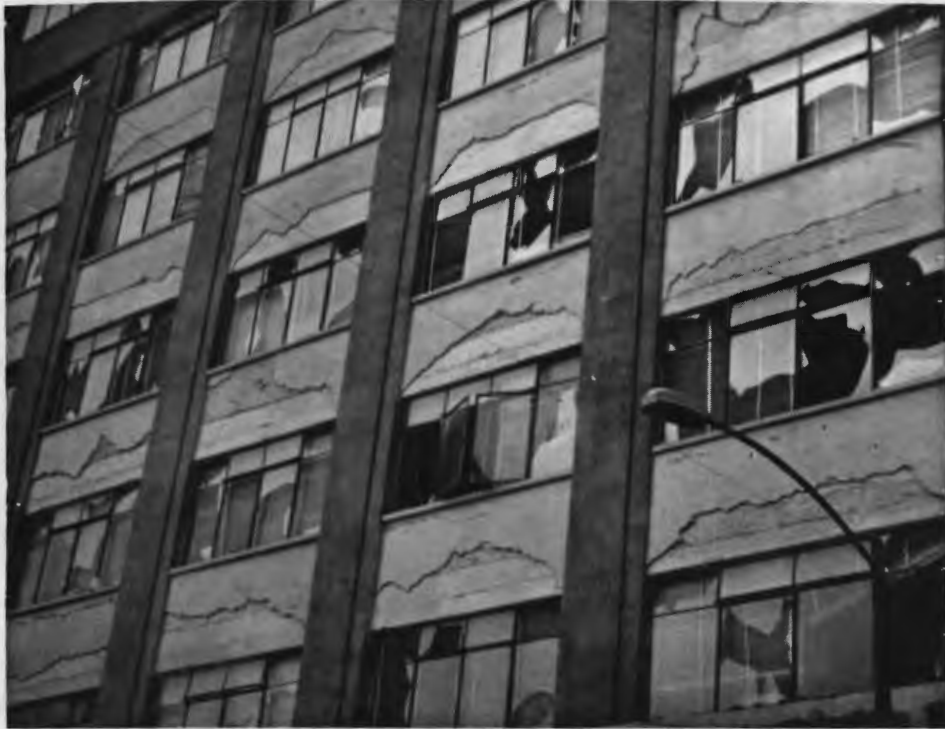
Building near Regis Hotel -- glass and stucco spandrel cracking
