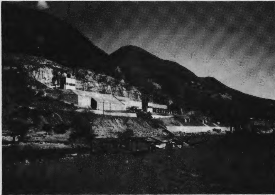
photo: EQE, Inc.
