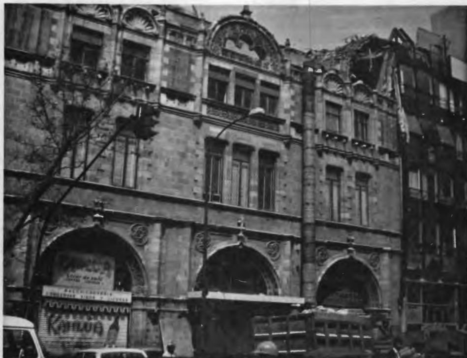
Undamaged old masonry building. Next door is newer office building with upper floor collapse
