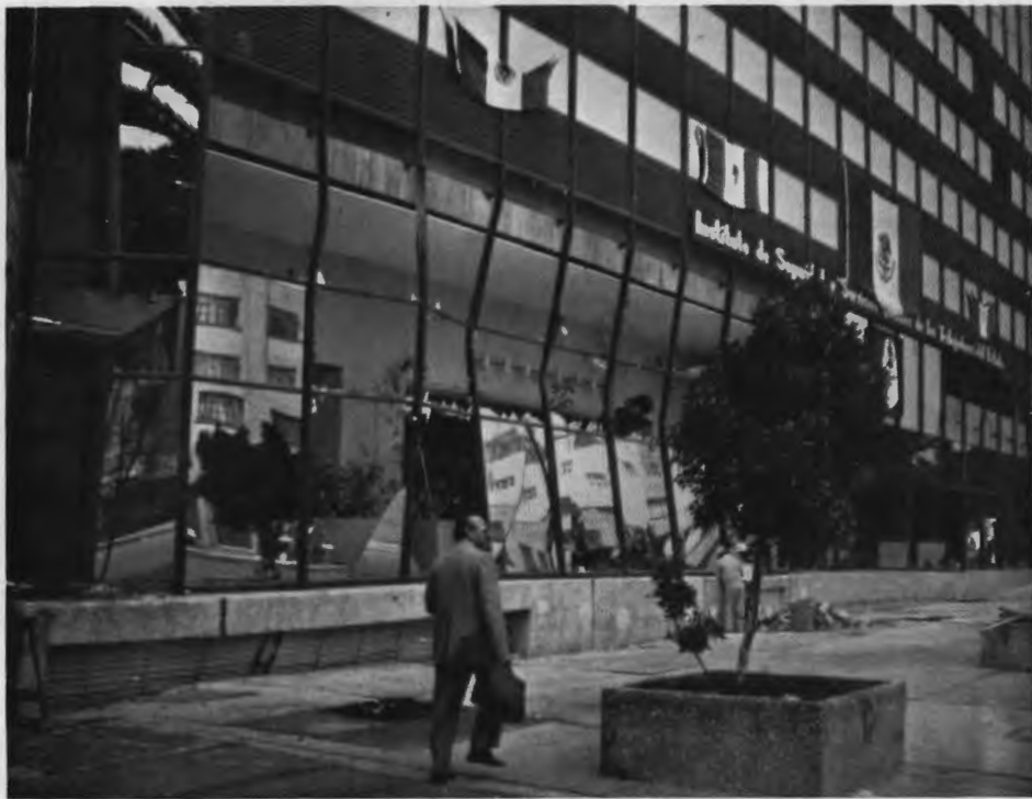
Distorted glass framing
