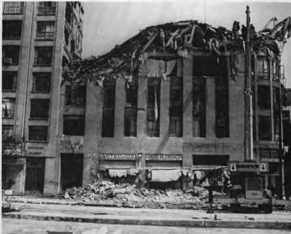
Older concrete building -- upper floor collapse
