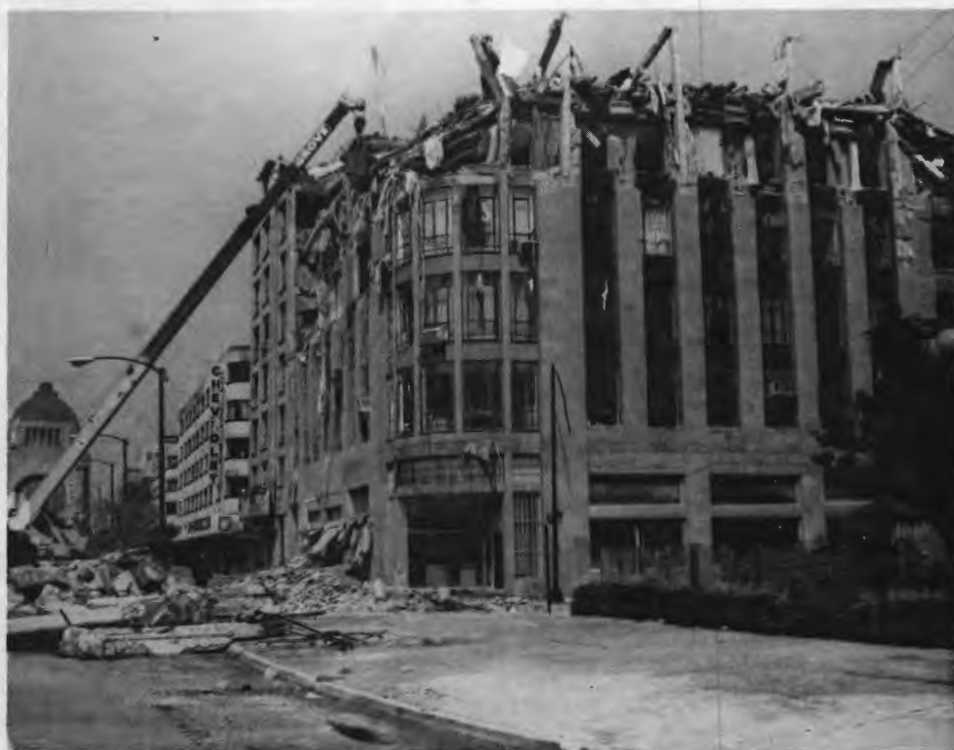
Older concrete building -- upper floor collapse
