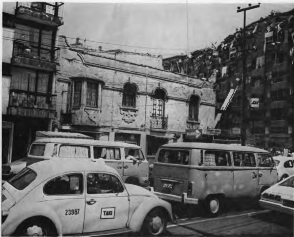
Intact old masonry building. Damaged government office building in background -- top floor collapse.
