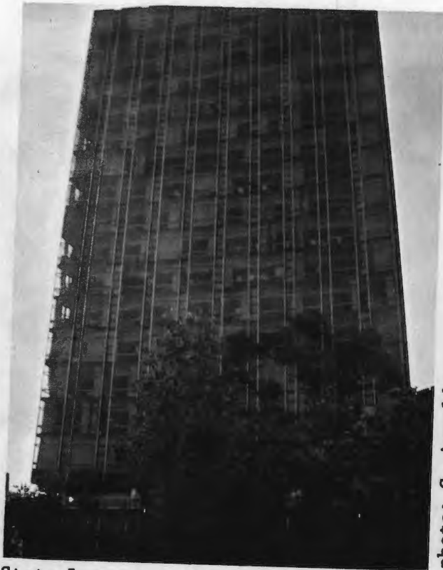
State Lottery building -- undamaged. This steel frame structure is located 1 block from Regis Hotel.
