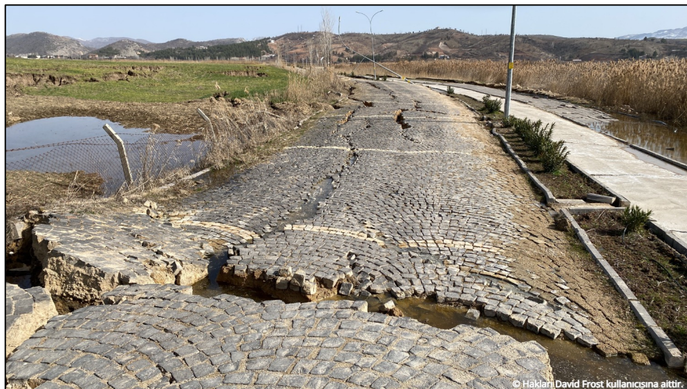
Lateral spreading and subsidence observed in Gölbaşı-Adiyaman adapted from Cetin et al. (2024)
