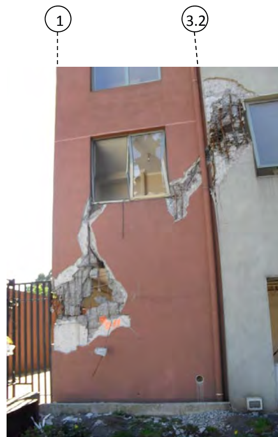
CM building: propagation of damage between stories
