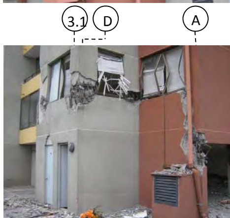
CM building: propagation of damage between stories
