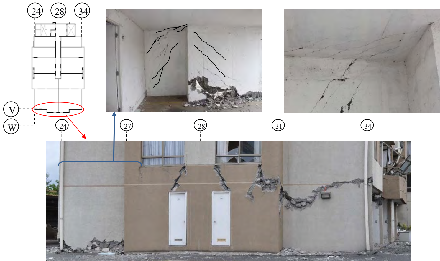
PdR building: damage propagation
