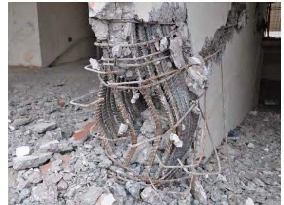
Typical confinement detail
