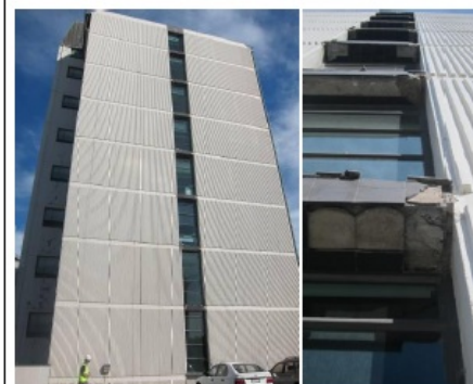
Detail 3: Minimal damage at the facade precast panels (except for local crushing at the slab-window region).
