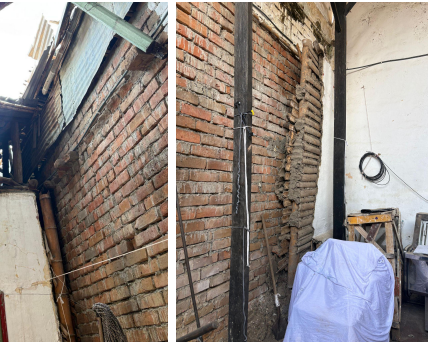
Damages in a wattle and daub ( bahareque in Spanish) building located in la Victoria, Valle del Cauca, Colombia. Photos: Jorge Archbold (2026). [11]
