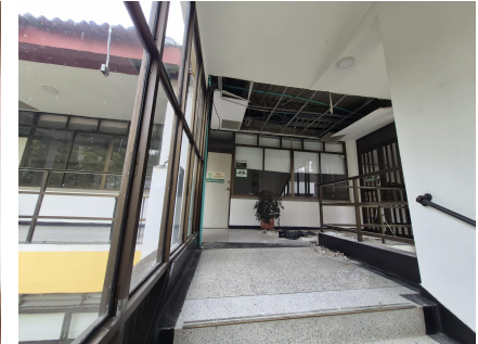
Damage in non-structural elements (infill walls and ceilings) in a building at Universidad Católica de Pereira, Risaralda. Photos: Raul Rincon (2026).[13]
