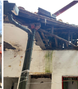
Damages in a wattle and daub ( bahareque in Spanish) building located in la Victoria, Valle del Cauca, Colombia. Photos: Jorge Archbold (2026). [11]
