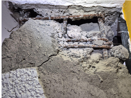
Out-of-plane failure of the façade wall, damage to infill walls, and structural damage to one column in a building at Universidad Católica de Pereira, Risaralda. Photos: Raul Rincon (2026). [12]
