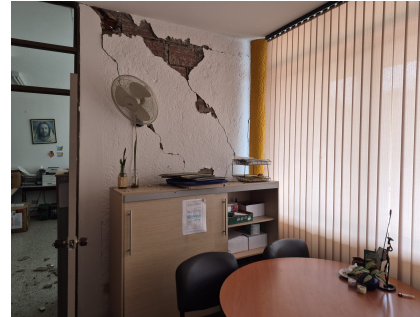
Damage in non-structural elements (infill walls and ceilings) in a building at Universidad Católica de Pereira, Risaralda. Photos: Raul Rincon (2026).[13]
