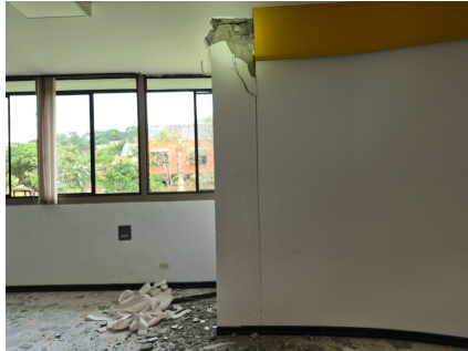
Out-of-plane failure of the façade wall, damage to infill walls, and structural damage to one column in a building at Universidad Católica de Pereira, Risaralda. Photos: Raul Rincon (2026). [12]
