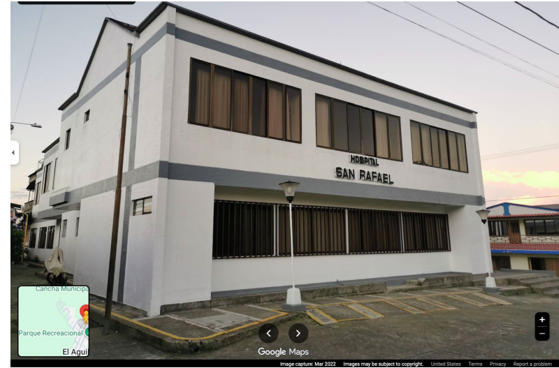
Front view of the San Rafael Hospital building before the earthquake, El Águila, Valle del Cauca region
