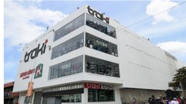
Commercial building damage. Edilson Gamez / Getty Images Building status: yellow.
