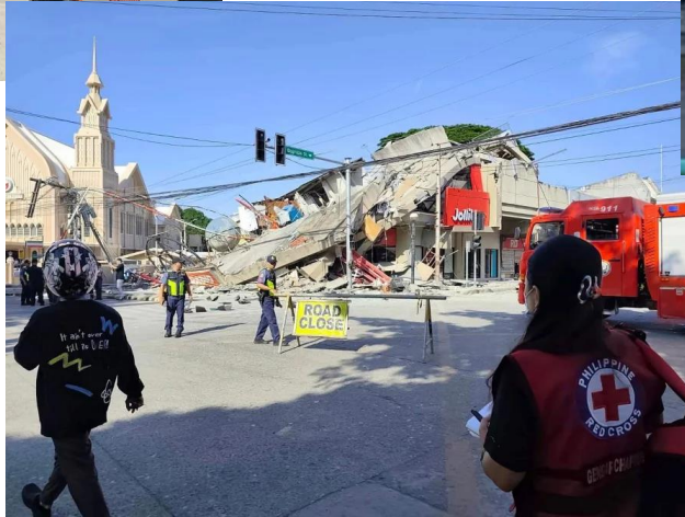
Philippine Red Cross at collapsed restaurant building in General Santos [8]
