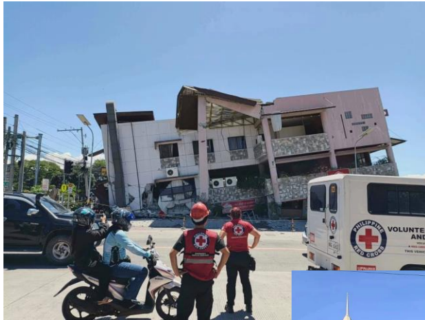
Philippine Red Cross at collapsed commercial building in General Santos [8]
