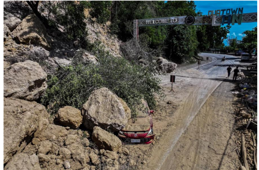
A drone shot shows a landslide following the magnitude 7.8 quake, in Barangay Kapatan, Glan, Sarangani province, southern Philippines, June 10. REUTERS/Adrian Portugal [5]
