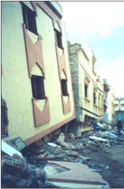
Figure 8. First-story collapse of several buildings (photo: Youd).
