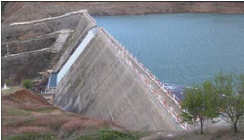
Figure 6. Joumoua Dam, a roller-compacted concrete structure completed in 1990, was undamaged by earthquake shaking (photo: Chraïbi).
