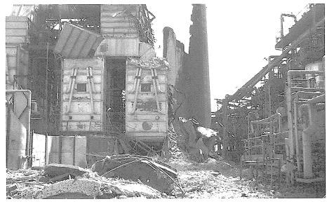
**Figure 15** - Collapsed 90-meter reinforced concrete stack at the Tupras refinery caused extensive damage and fires. (Photo: Johnson)
