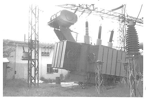
**Figure 13-** Damage to transformer in Izmit-2 substation. Tilting due to movement of support. (Photo: Basoz)
