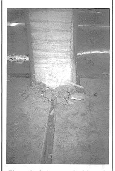
Figure 3 - Column pushed through the floor slab and tilted due to 0.5 right-lateral fault displacement. Coiumn underwent ductile deformation without losing significant axial load capacity. (Photo: Youd)
