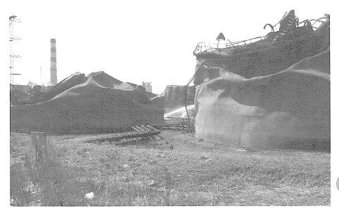
**Figure 17-** Tanks destroyed by out-of-control fire in the Tupras refinery tank farm. (Photo: G. Johnson)
