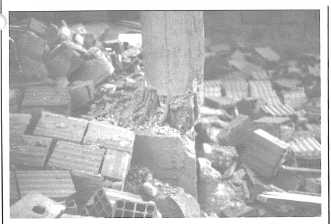
Figure 8 - Typical weak-axis column hinging.
