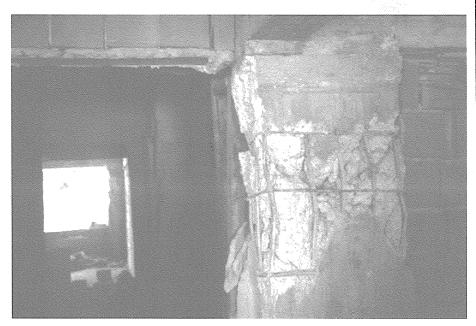
Figure 9 - Typical strong-axis column shear failure.
