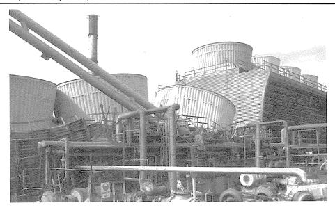
**Figure 16** - Collapsed wooden cooling towers at the Petkim petrochemical plant. Instrument at the site measured peak horizontal acceleration at 0.32g. (Photo: Johnson)
