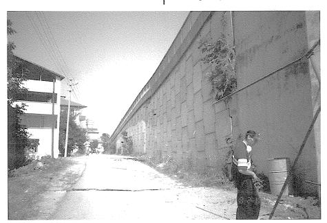
**Figure 5 -** Mechanically stabilized earth wall within a few meters of the primary fault rupture. Although subjected to differential settlement, it suffered only minor damage. (Photo: Youd)
