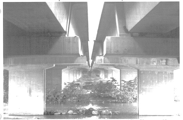
Figure 11 - The east (left) and westbound bridges over the Sakarya River. Note shifting of the spans and the unseating of the bearings in the westbound bridge. The bearings on the eastbound bridge have partially "walked out," but not unseated.
