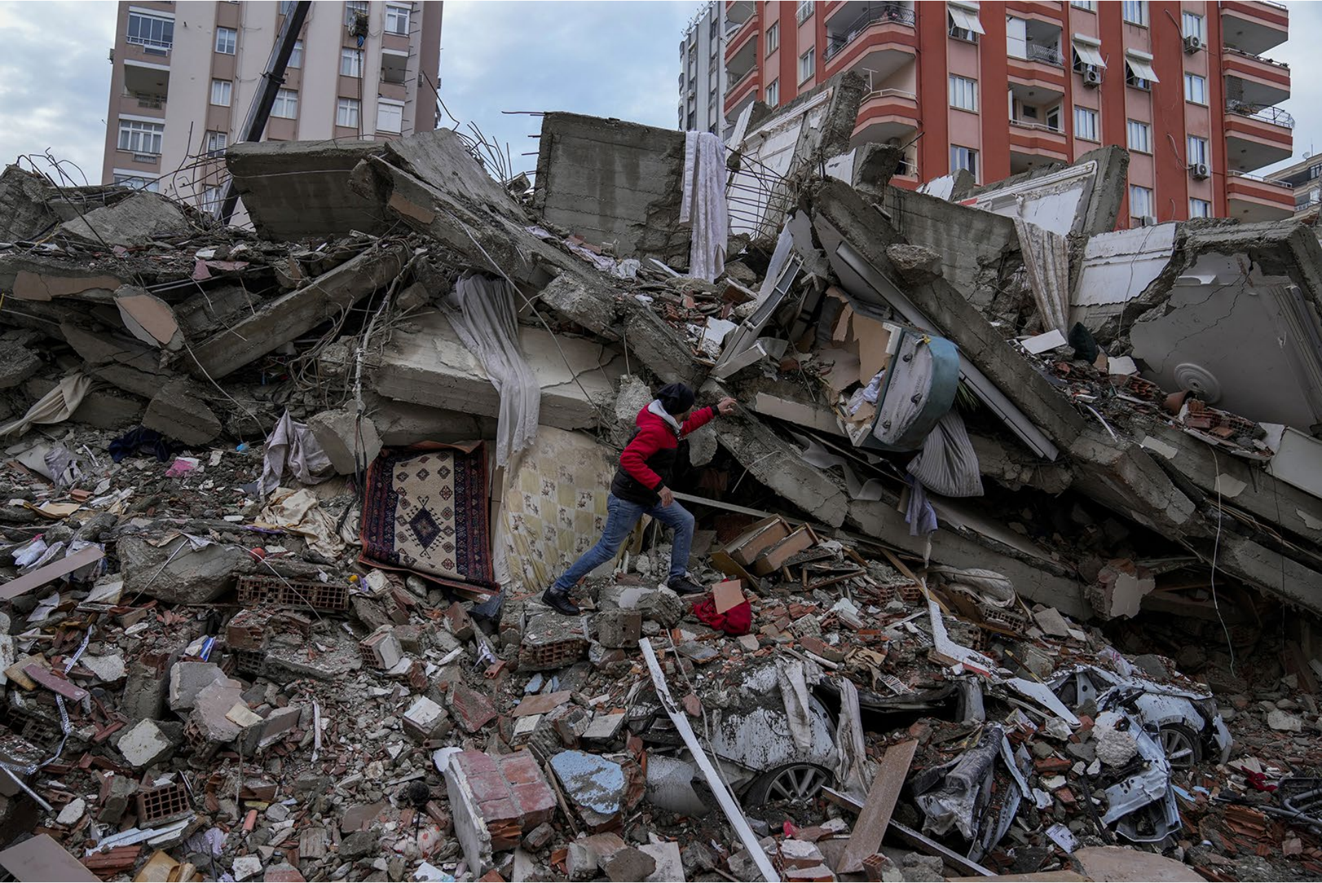
Rubbles of a destroyed building in Adana, Turkey, Monday, Feb. 6, 2023. Source: AP Photo/Khalil Hamra
