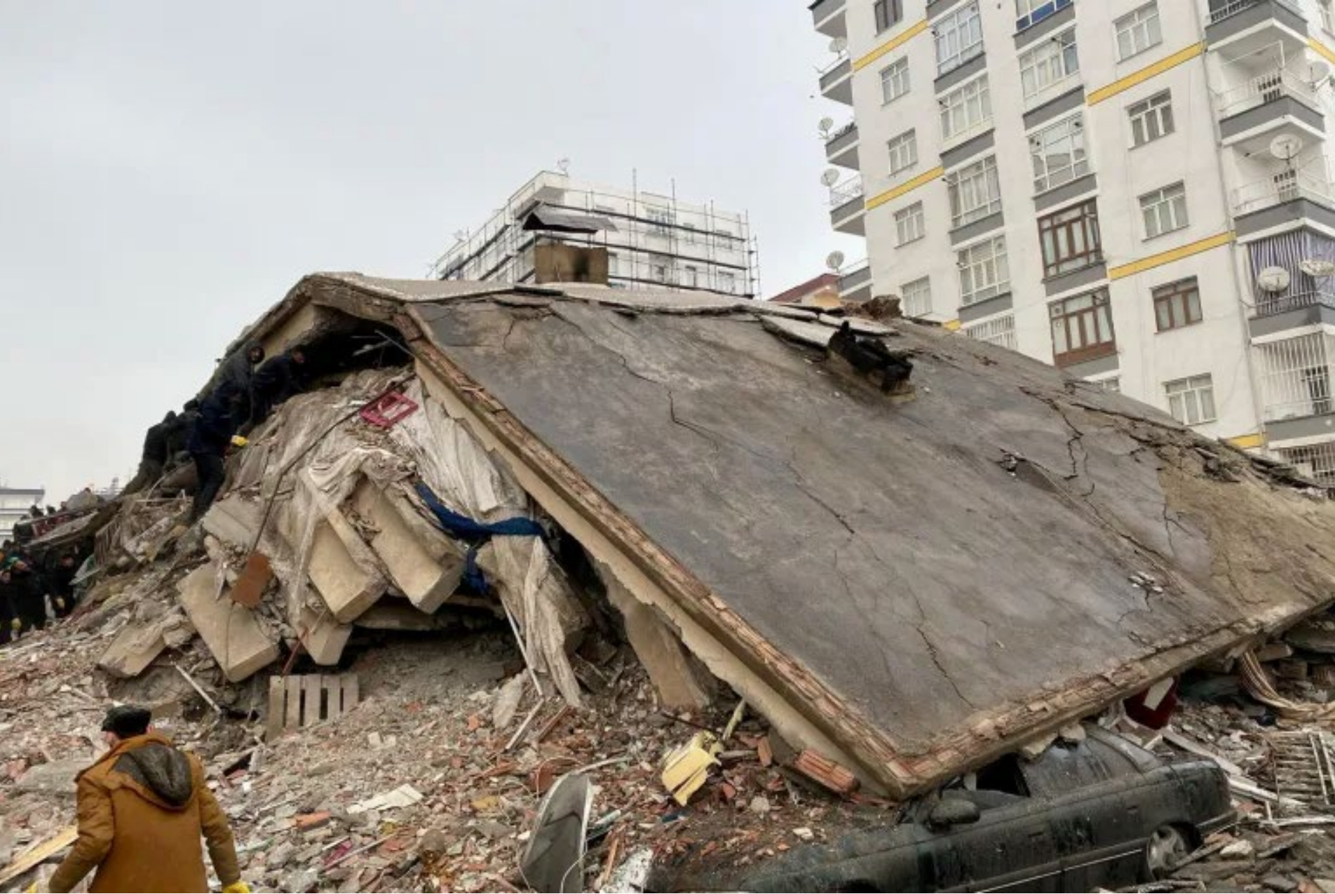
People search through rubble following an earthquake in Diyarbakir, Turkey, February 6, 2023 [Sertac Kayar/Reuters]
