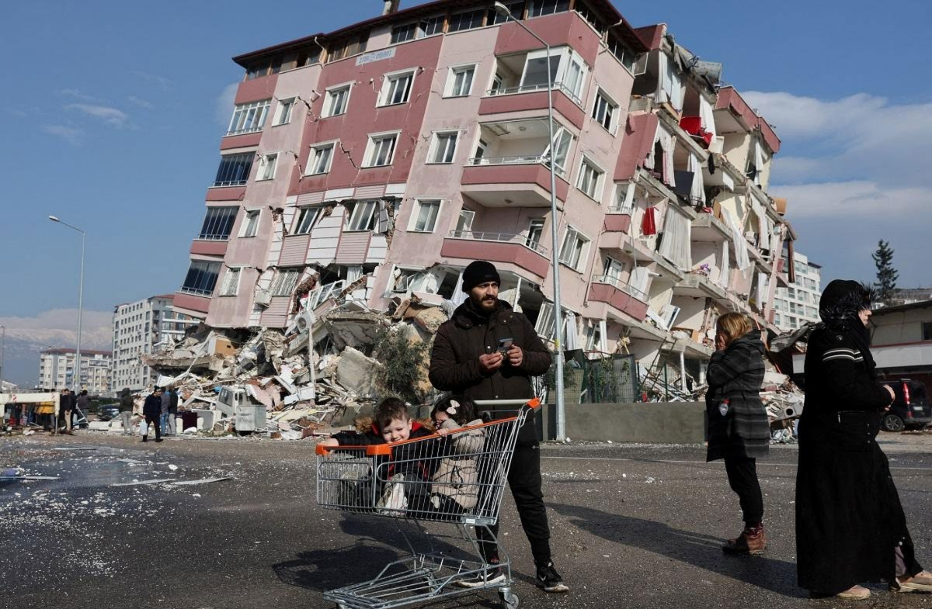
A collapsed building in Hatay, Turkey, February 7, 2023. (Photo: REUTERS/ Umit Bektas/ File Photo)
