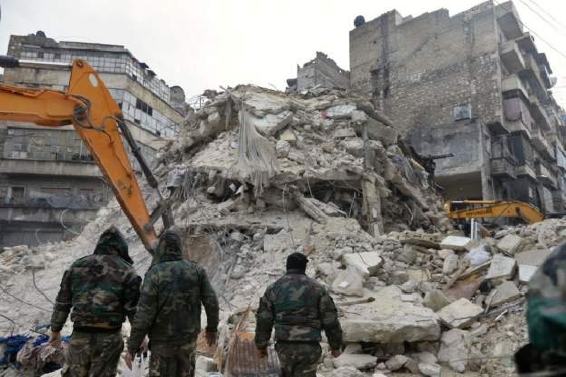
Rescue teams search for victims and survivors in the rubble of a collapsed building in the Syrian city of Aleppo (Source: BBC, AFP)
