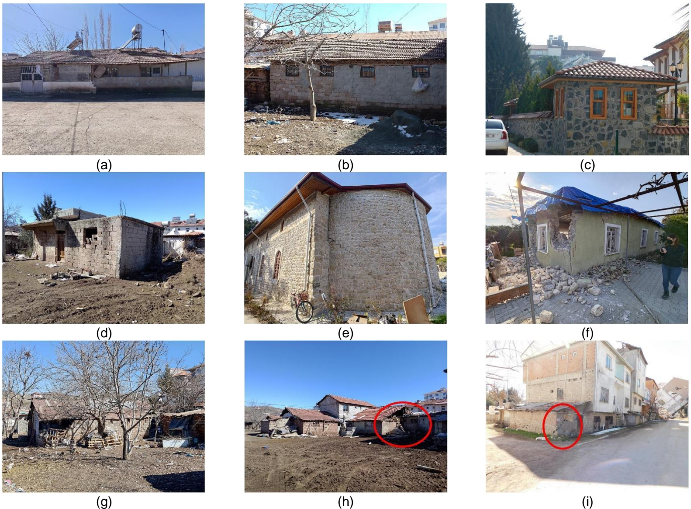
Figure 4-9 (a) to (c) essentially intact or slightly damaged masonry buildings, (d) and (e) moderately damaged masonry buildings, (f) to (h) severely damaged masonry buildings, (i) a pure sliding mode of failure mechanism of a brick wall.
