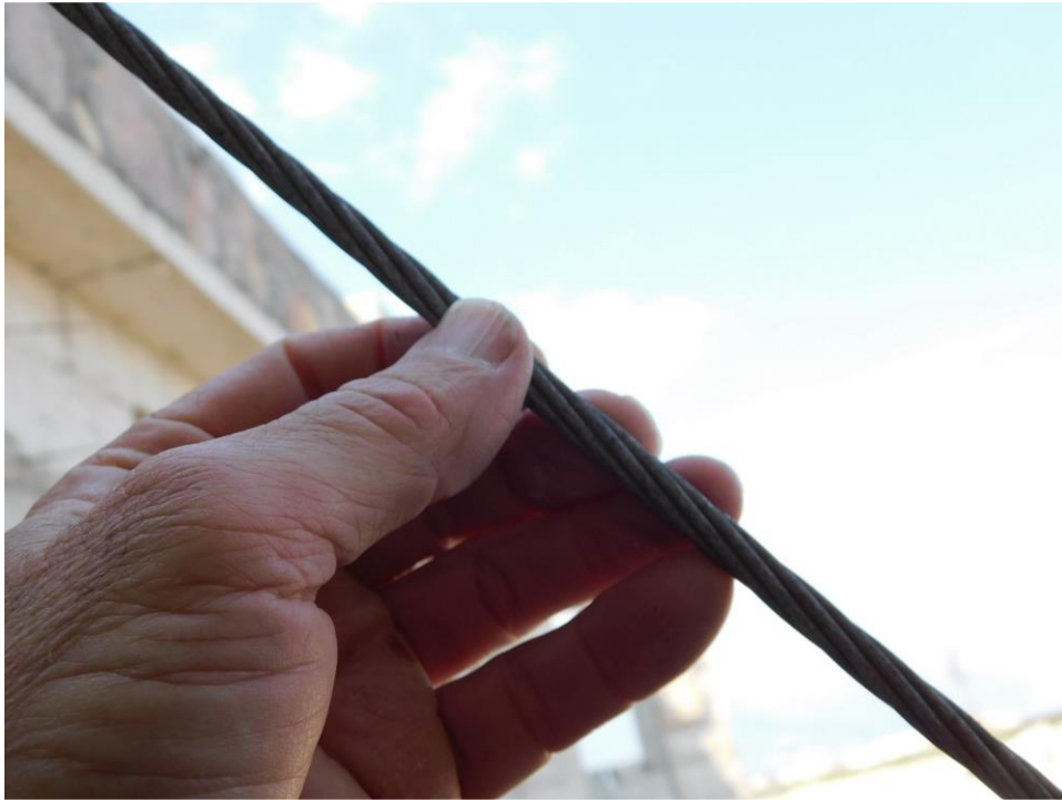
Figure 5-22 Close-up view of prestressing cable near end of precast girder, Bridge 2
