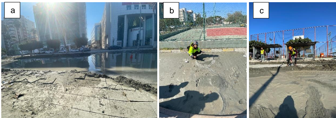
Figure 3-6 Liquefaction manifestations on Ataturk Boulevard near Tennis Courts (~ 36°35'26.95"N/ 36° 10'28.39"E): a) water accumulation and sand boils; b) sand boils; c) ground settlement.
