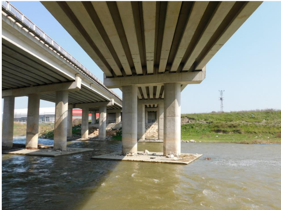
Figure 5-13 Overall view from under Bridge 2
