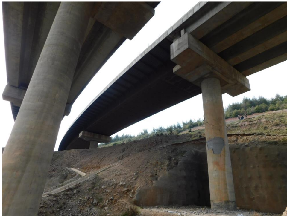
(b) Looking toward opposite abutments of adjacent bridges
