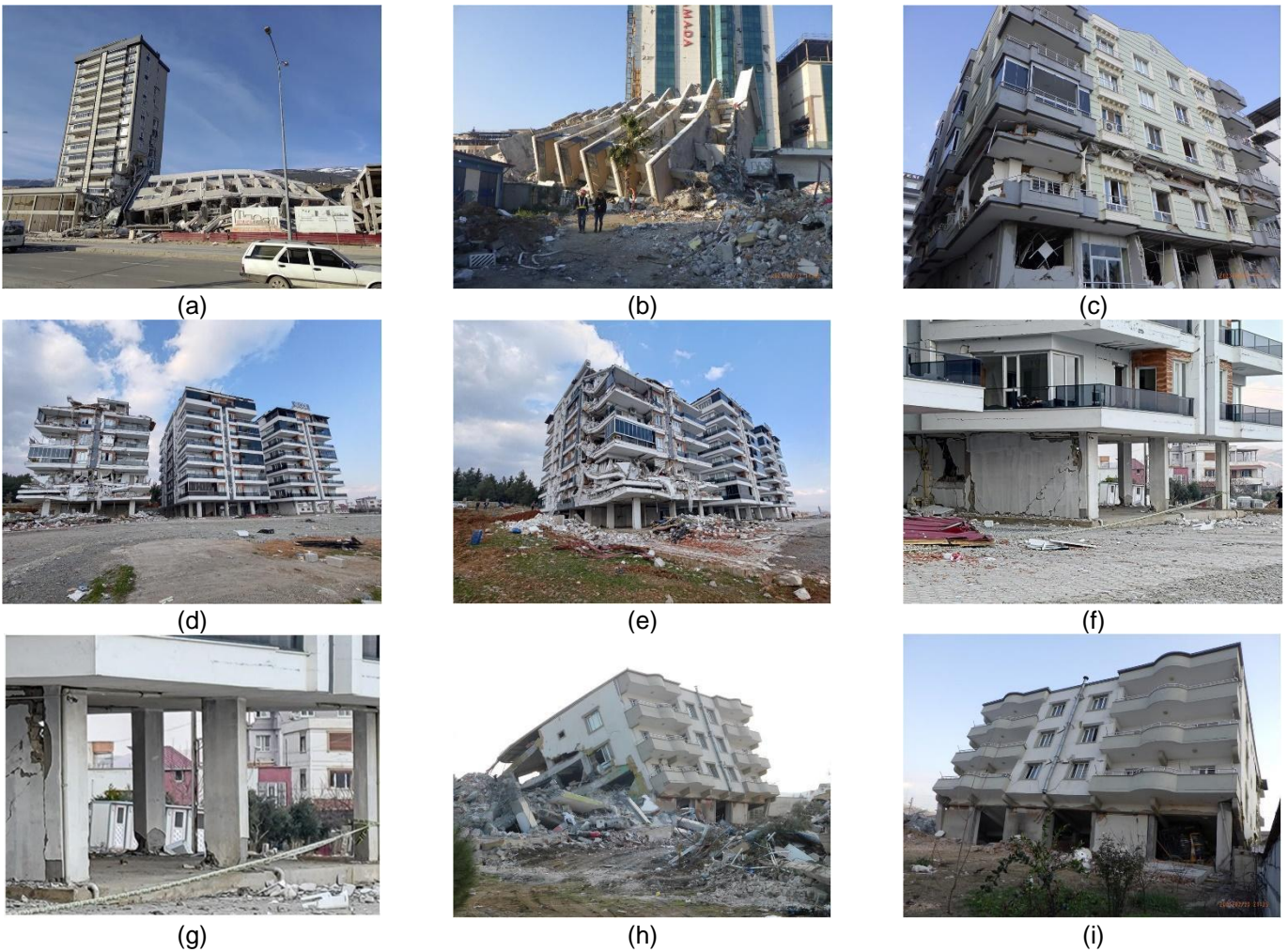
Figure 4-3 (a) and (b) lie-down collapsed buildings, (c) a building with pancaked third story, (d) and (e) three similar buildings with different damage states, (f) close-up photograph of the first story of the right building, (g) bi-directional and one-directional plastic hinges, (h) and (i) a knee-down collapsed building.
