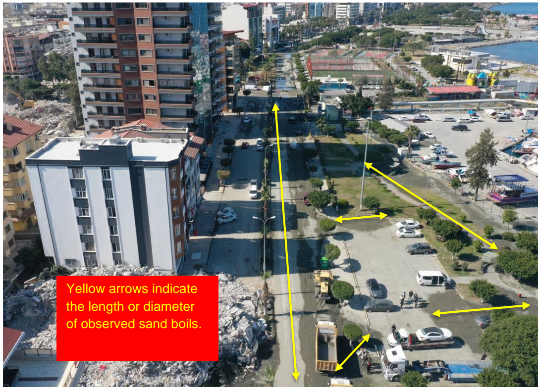
Figure 3-5 Liquefaction manifestations (sand boils) on Ataturk Boulevard (~ 36°35'26.86"N/ 36° 10'40.39"E)
