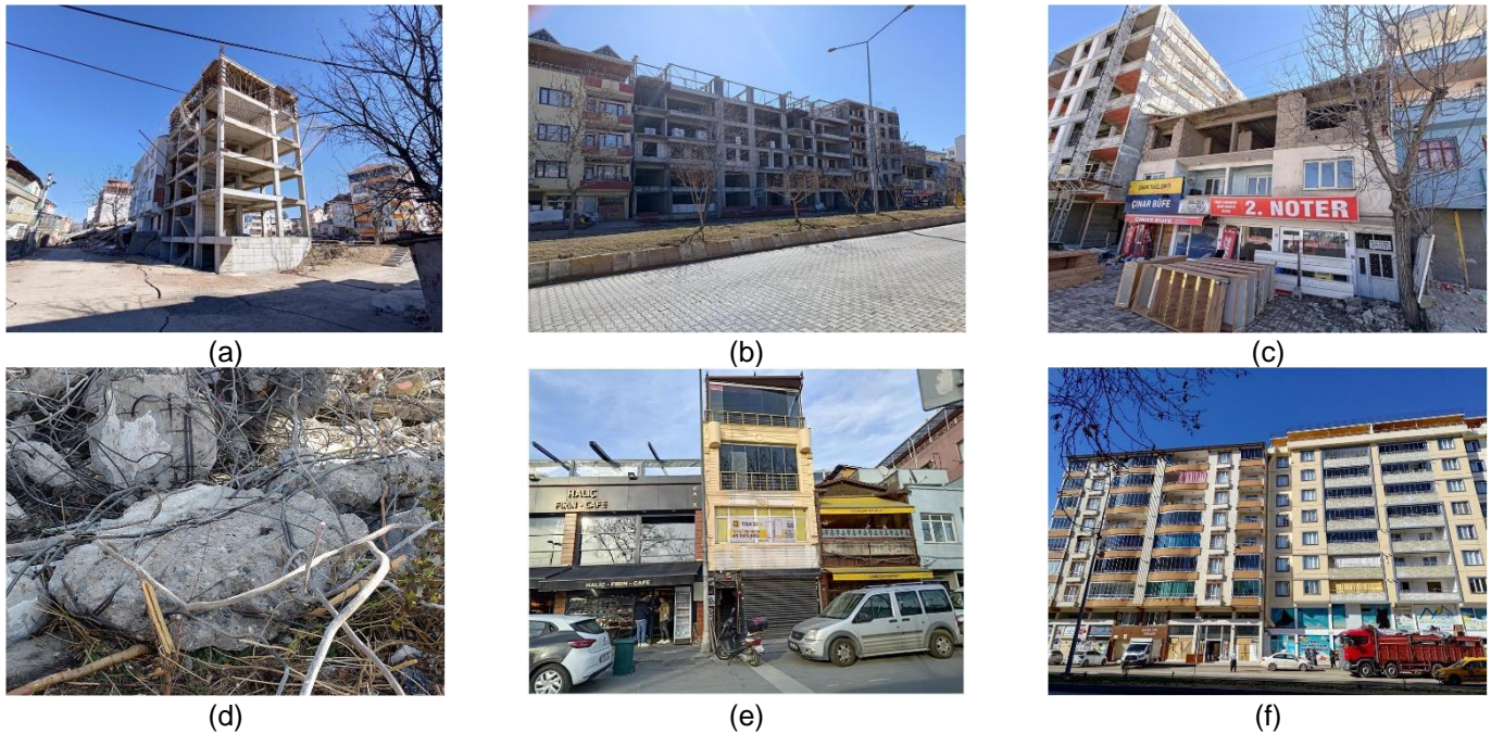
Figure 4-2 (a) and (b) two buildings with different construction practices, (c) a building with an added third story, (d) poor concrete and plain reinforcement, (e) and (f) no separation between buildings.
