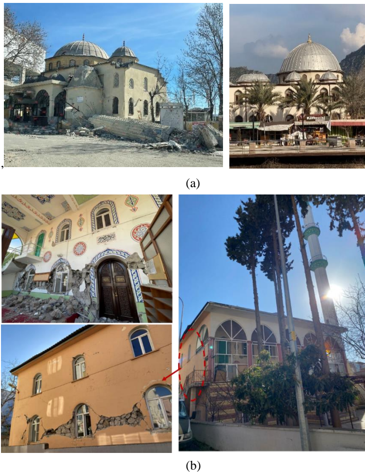
Figure 7-2 Damage of Mosques (a) Haci Murat Mosque in Kahramanmaras, (b) Merkez Cumhuriyet Mosque in Pazarcik
