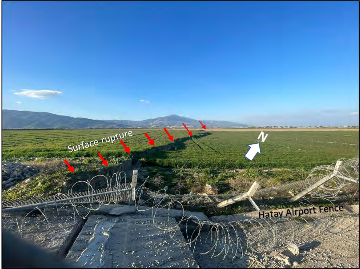
Figure 2.7. February 6, 2023 M7.8 Kahramanmaraş earthquake surface rupture at the Hatay Airport north fence. Note the left-stepping en-echelon left-lateral surface rupture with down-to-the-east vertical component. Lat/Long: 36.366992°N, 36.279822°E. Photo taken February 15, 2023.
