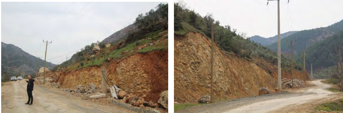
Figure 7.31. Rockfall damaged concrete distribution poles, replacement wood poles (near ID 141).
