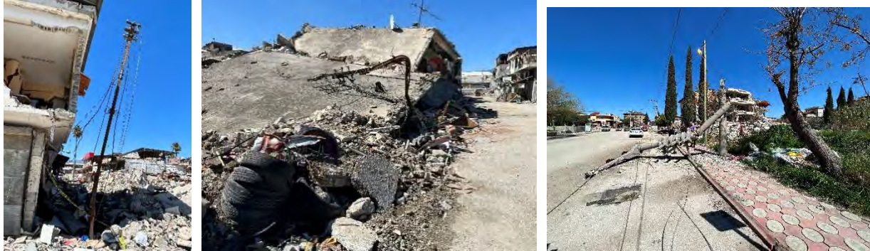
Figure 7.30. Distribution overhead structures damaged by debris (Antakya).
