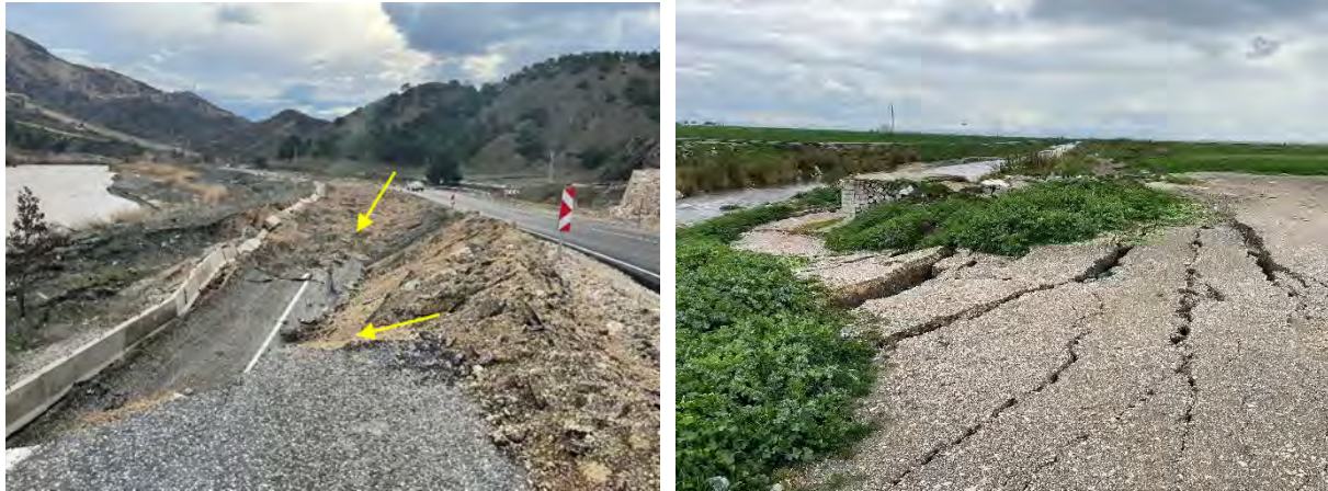
Figure 7.9. Embankment and roadway failure near a dam located (left, ID No. 83 in Appendix A) and near a bridge (right, ID No. 45 in Appendix A).
