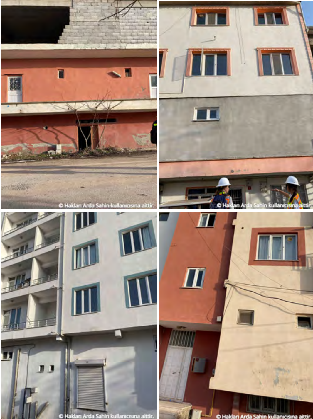
Figure 4.9. Top left: coordinates -37.78994, 37.65102, no tilt, vertical Settlement 20 cm, GF3, D1. Top right: coordinates -37.79000, 37.65115, no tilt, vertical settlement 30cm, GF3,D0. Bottom left: coordinates- 37.79003, 37.65122, no tilt, settlement 99 cm, GF3, D1. Bottom right: coordinates- 37.78978, 37.65076, 1 degree tilt, 10 cm settlement, D0, GF2.
