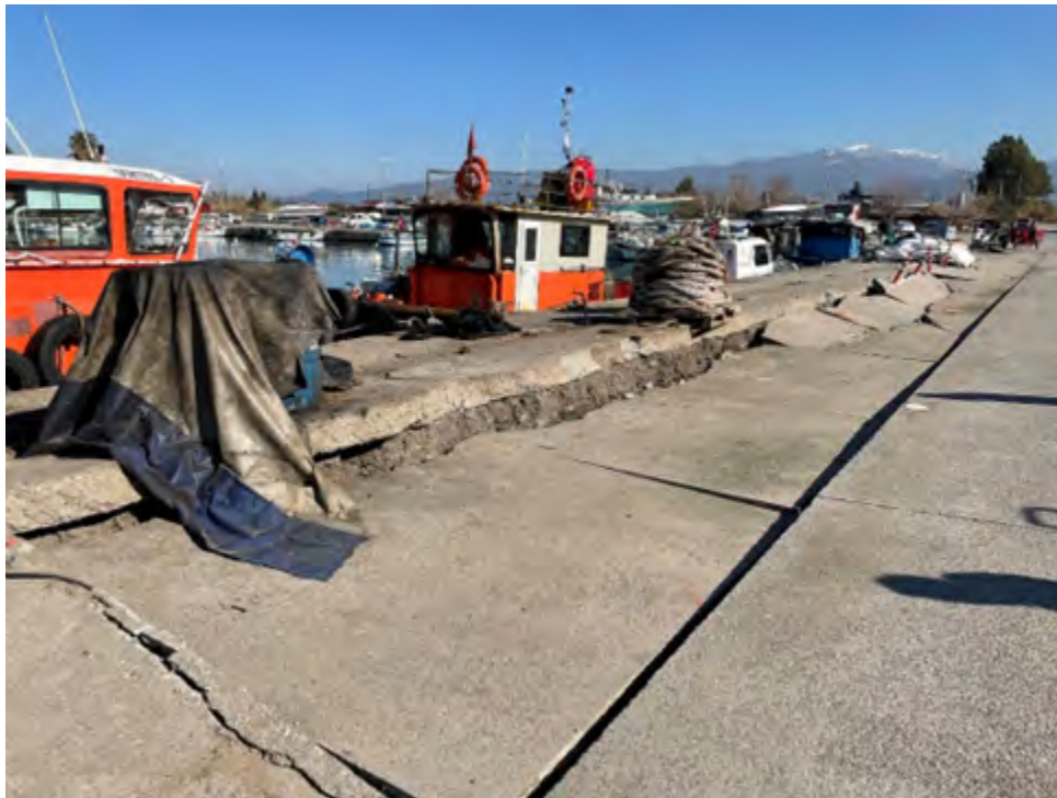
Figure 4.56: Liquefaction-induced lateral spreading and surface manifestation of liquefaction at Fisherman's Wharf, Dörtyol-Hatay (36.820771 N, 36.173860 E)
