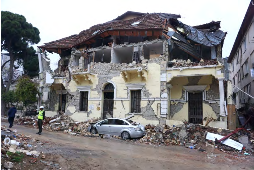
Figure 5.41. Damage to the unreinforced masonry building housing the Antik Beyazit Hotel.
