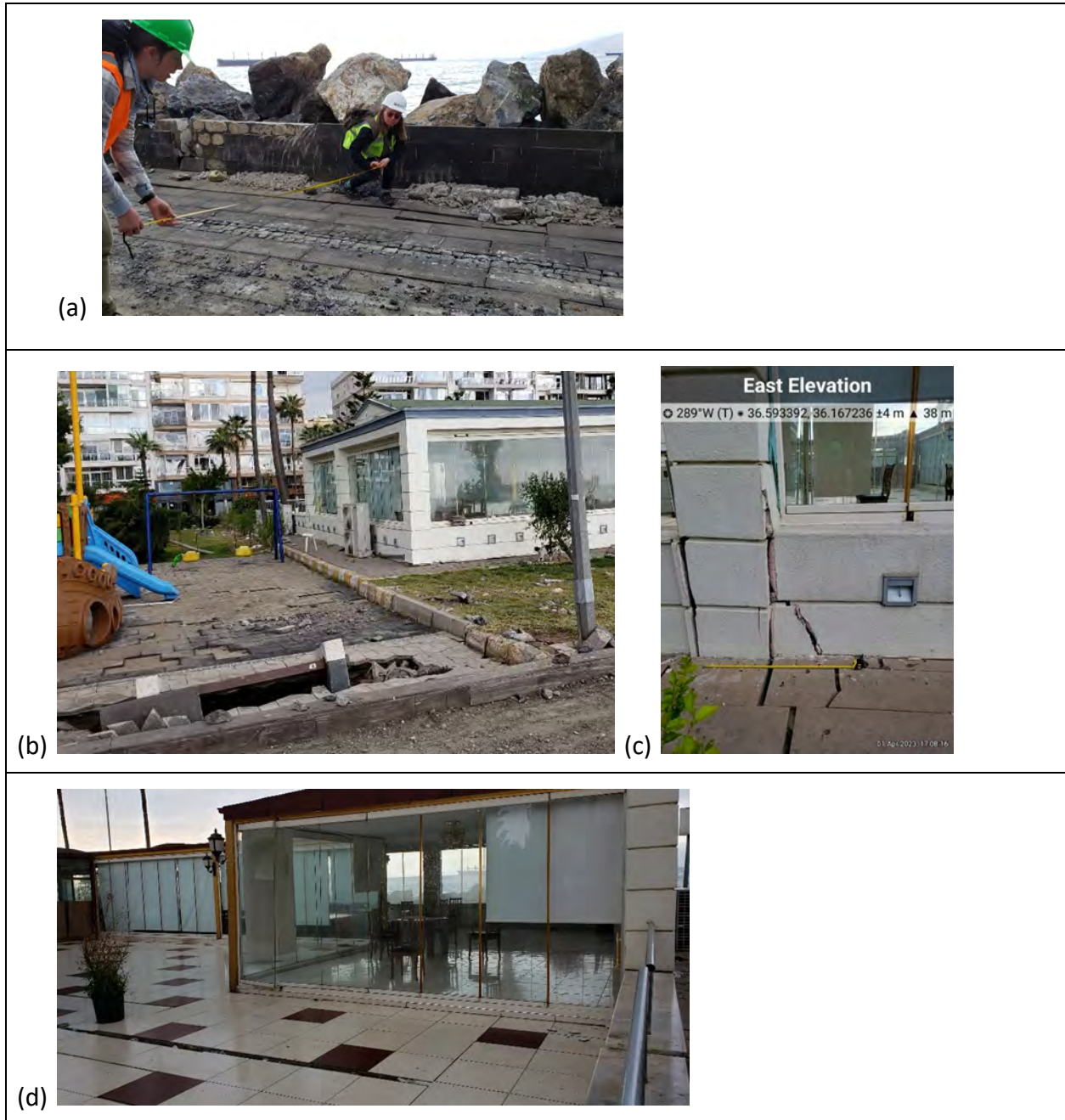
Fig 4.30. Photos of lateral spread LS-2 taken April 1, 2023: (a) seawall at start of LS-2 (N36.59367°, E36.167191°), (b) sunken park bench and spreading along eastern wall of Doğan restaurant patio (N36.59367°, E36.167191°), (c) cracks near column at southeast corner of patio (N36.593392°, E36.167236°), (d) cracking along back of patio (N36.59345°, E36.16712°).
