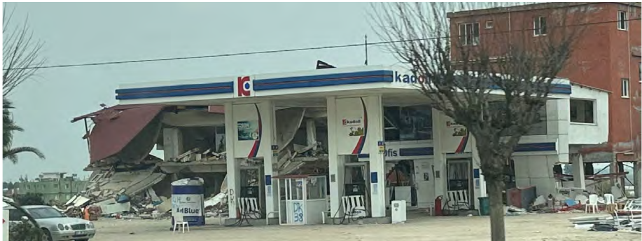
Figure 7.40. Example of petrol station in Antakya with standing canopy structure and heavily damaged one-story accessory building.
