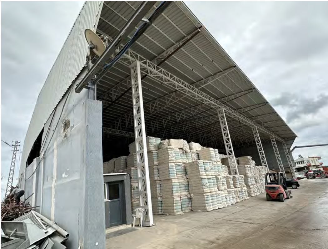
Figure 5.61. Good performance of steel frame industrial structure in Kırıkhan. Note the damage to the infill wall on the left side of the photograph.
