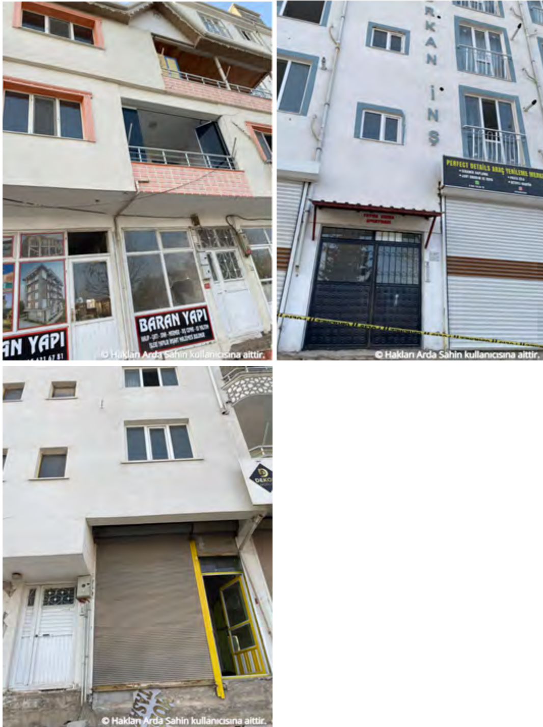
Figure 4.11. Top left: coordinates -37.78984, 37.65125, no tilt, vertical Settlement 20 cm, GF2, D1. Top right: coordinates -37.78996, 37.65139, 5° tilt, vertical settlement 28cm, GF3,D0. Bottom left: coordinates- 37.79014, 37.65161, 3° tilt, settlement 23 cm, GF3, D1.
