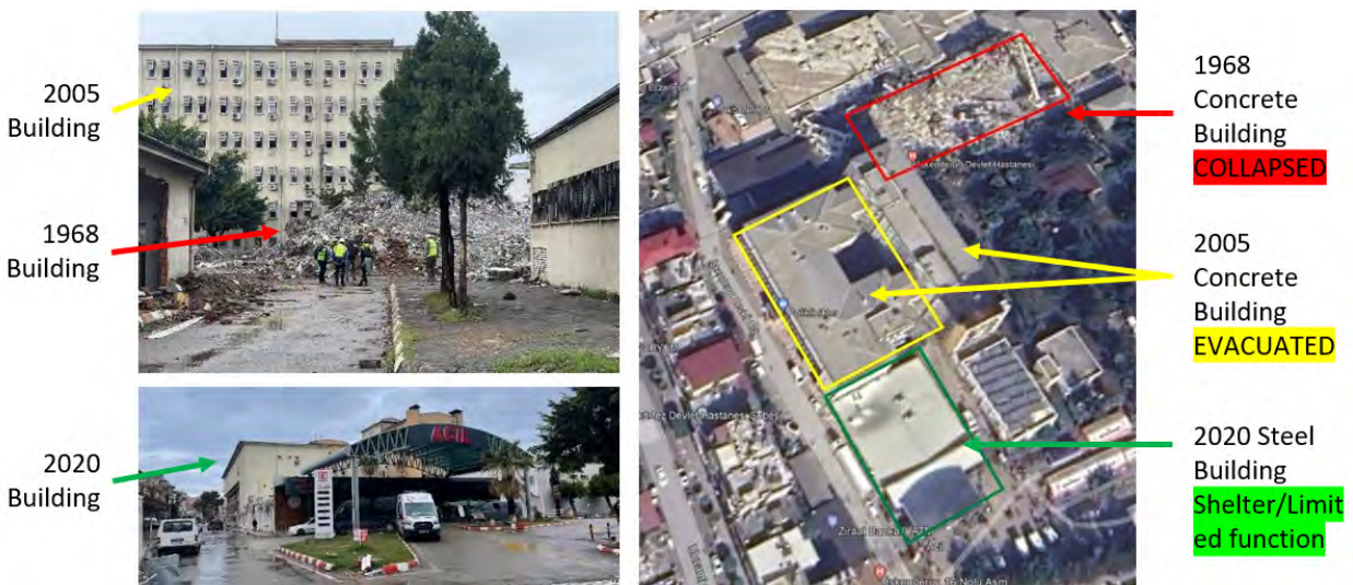
Figure 6.6. İskenderun Government Hospital as observed on March 15, 2023 (photos on right) , PGA = 0.28g, PGV = 55cm/s, This hospital contained multiple buildings constructed between 1968 and 2020. The 1968 building collapsed, the 2005 suffered extensive nonstructural damage and could not be occupied. All patients were relocated to the floor of the 2020 steel building before being transferred to other facilities.
