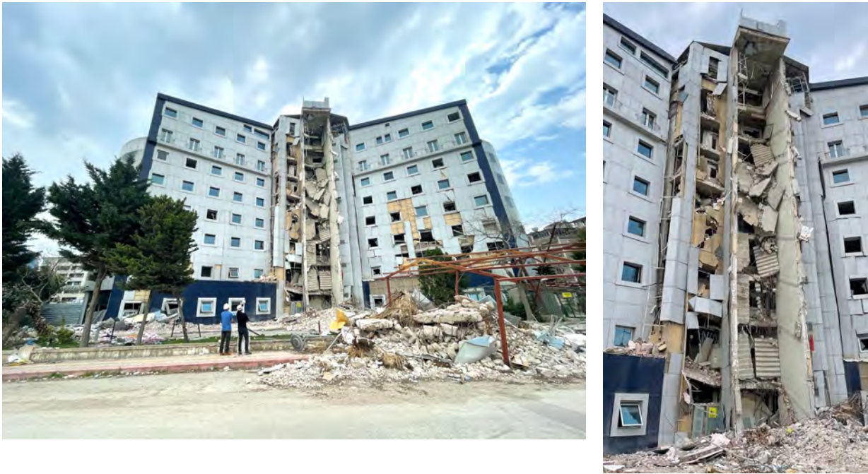
Figure 6.10 Collapsed egress stair Defne Private Hospital, Antakya, Hatay as observed on March 18, 2023. PGA = 0.98g, PGV = 132 cm/s.
