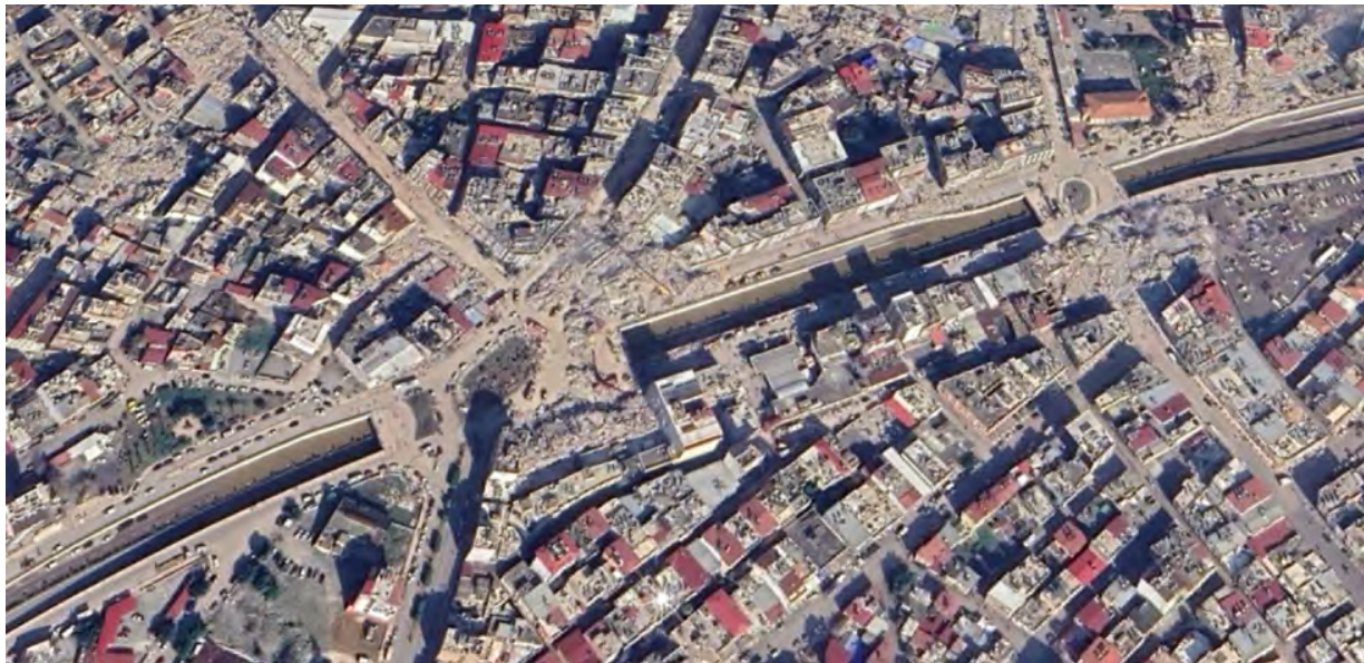
Figure 4.42. Image of u-box underpass in İskenderun, Hatay from Google Earth on 8-February-2023, showing flood water in the underpass.
