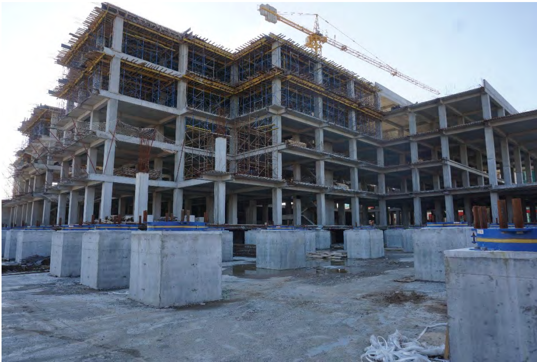
Figure 5.48. Base isolated hospital building under construction in Kahramanmaraş.
