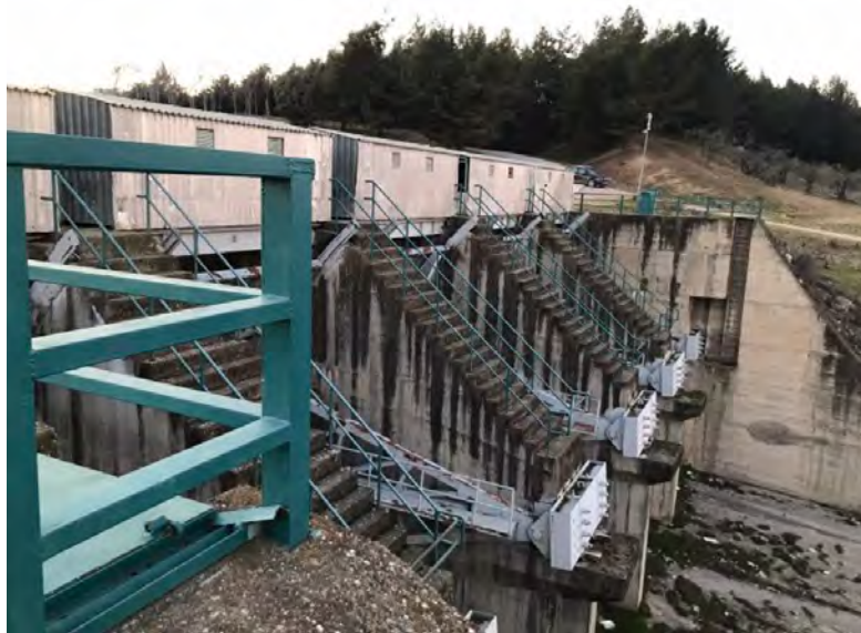
Figure 8.15. No observed cracking in the outlet structures.
