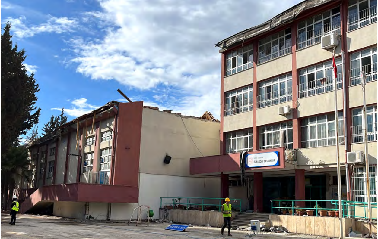
Figure 5.79. Collapse of wood-frame gable roof structure in a school building in Antakya.
