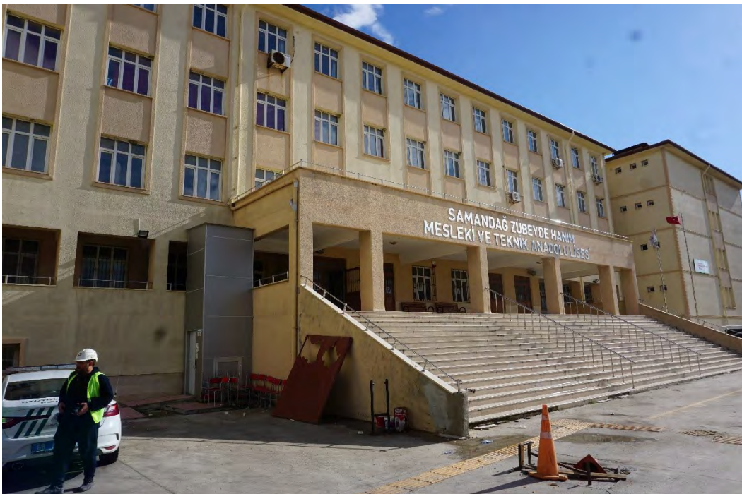
Figure 5.47. School building in Samandağ.
