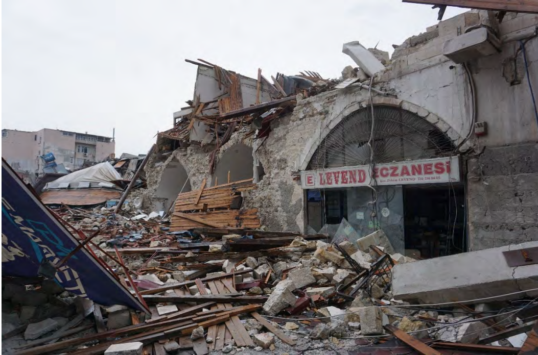
Figure 5.45. Collapse of the second story onto the first story at a multi-tenant commercial building.
