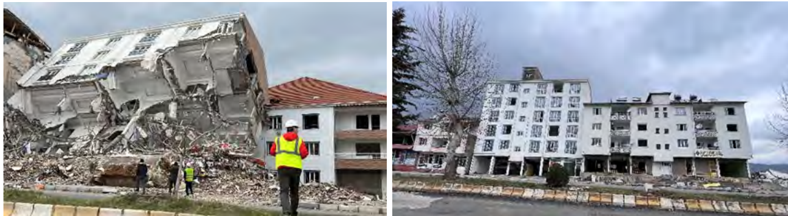
Figure 5.22. Overturning and tilting of structures due to liquefaction, İskenderun
