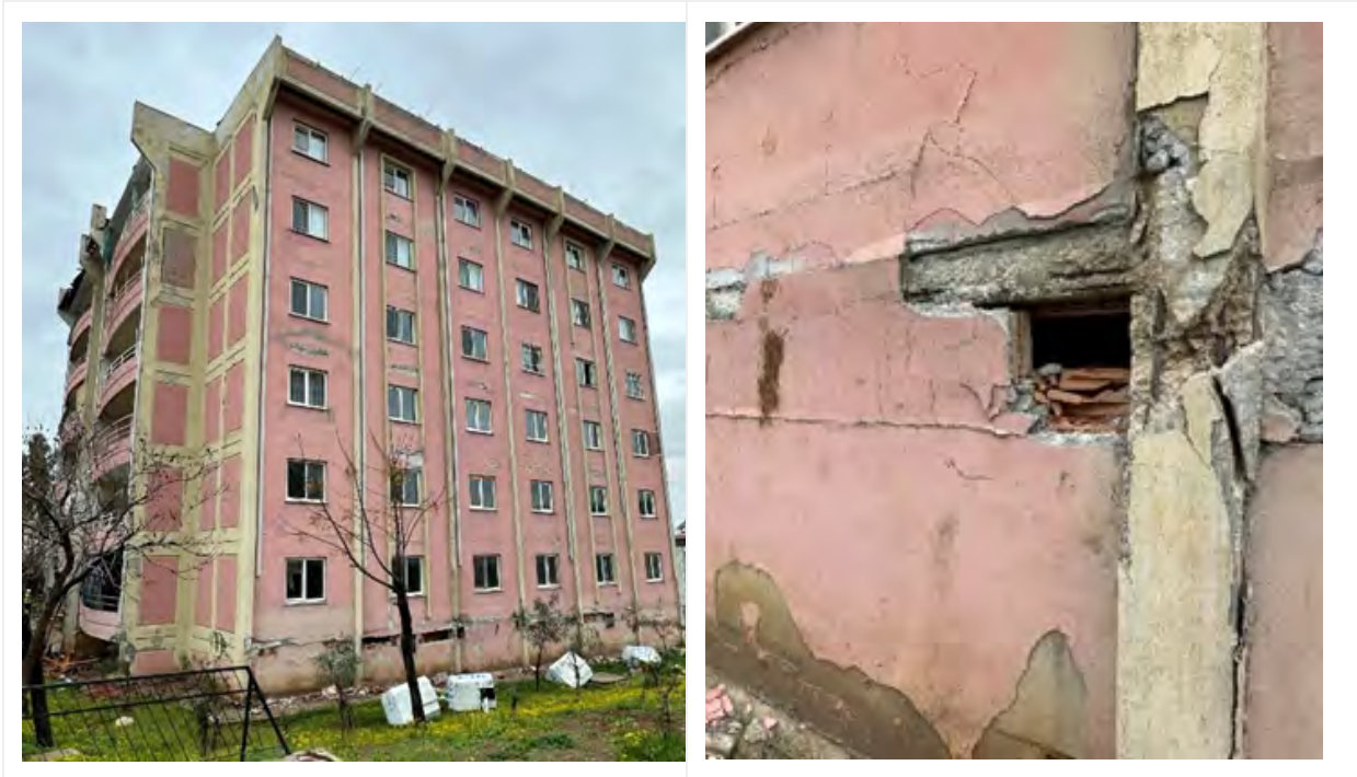
Figure 5.15: Localized short column effect induced by partial failure of masonry infill walls.
