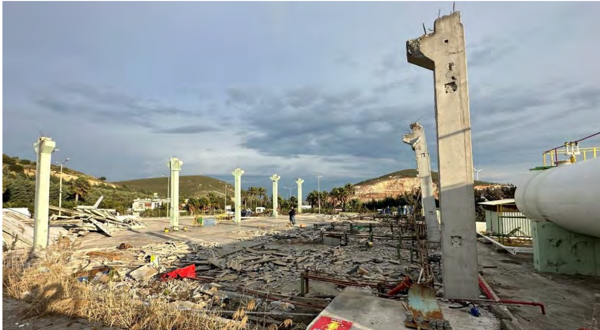
Figure 7.34. Collapse of precast production building at the Hasgaz plant west of Antakya.
