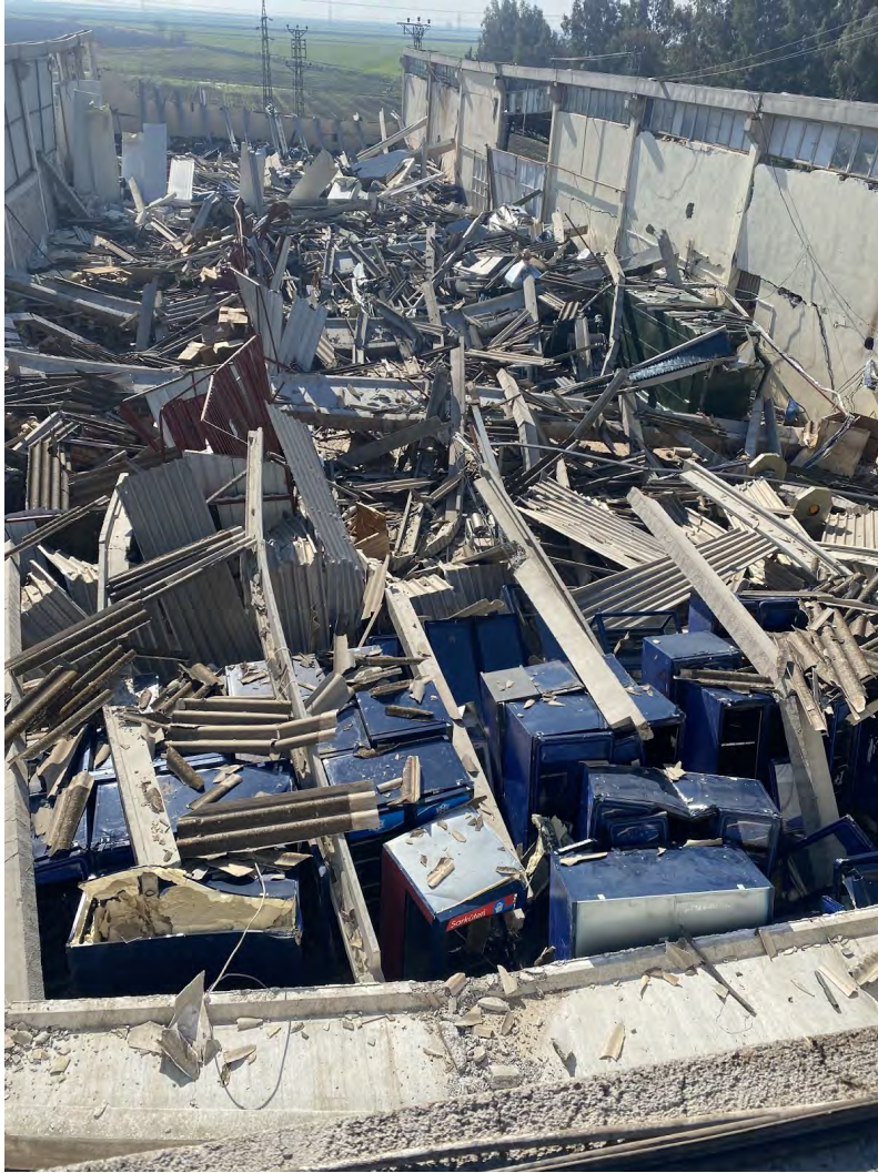
Figure 5.62. Remnants of precast concrete industrial building in Kırıkhan. The photograph was taken by the owner prior to the cleanup of debris.
