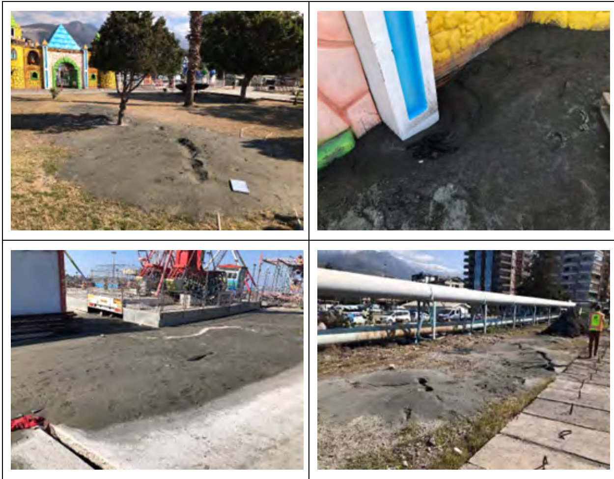
Figure 4.24: Liquefaction-induced ejecta in Atatürk Boulevard (36.591661 N, 36.175382 E).
