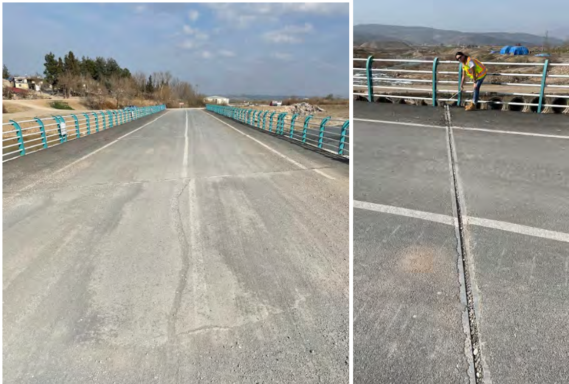
Figure 4.64. Isolated bridge near Kılılı (37.4123, 36.9066) with good performance. Photos taken March 4, 2023.
