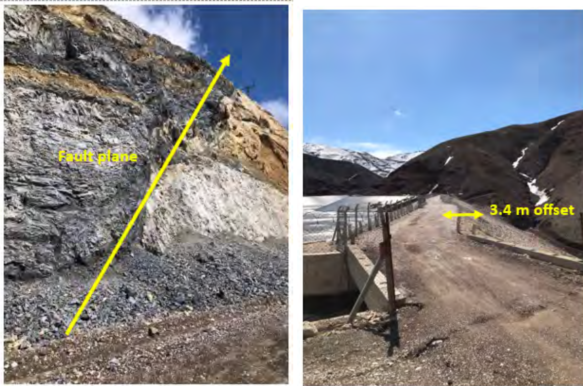
Figure 8.20. Left image shows the faulting in a cut near the dam. Right image shows evidence of the 3.4 meters of offset in the dam embankment.
