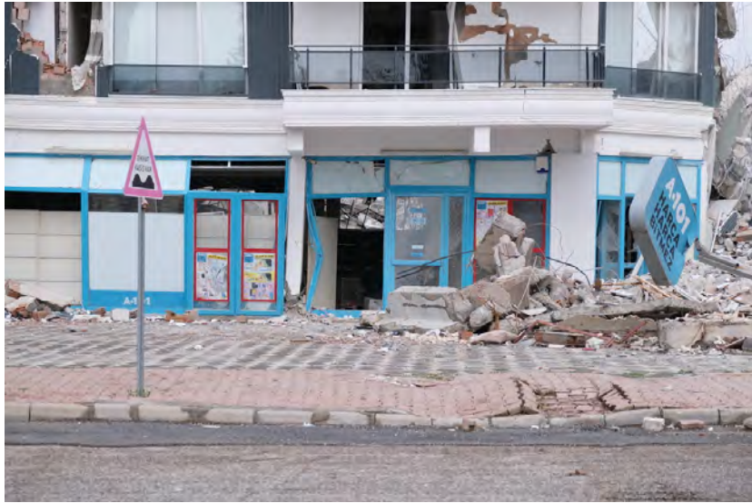
Figure 5.73. Failure of metal frame in storefront glazing due to structural damage in columns of a mixed use building near Adiyaman.
