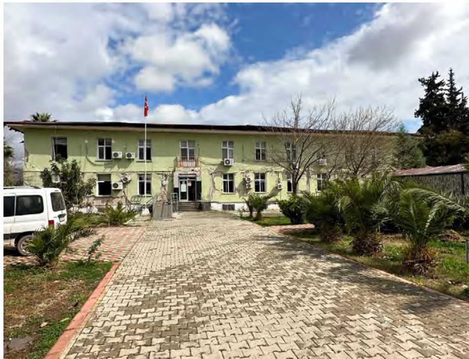
Figure 5.54. Courthouse building in Hassa.
