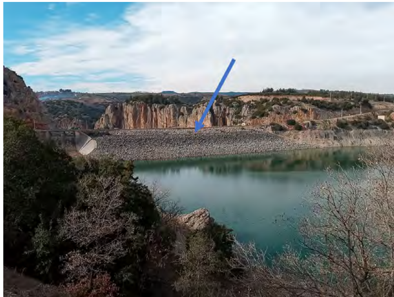
Figure 8.8. Arrow points to the midpoint of the dam where the largest crest deformations were observed. The highwater line (aka bathtub ring) as indicated by the black line shows a “swayback” response due to seismic compression.
