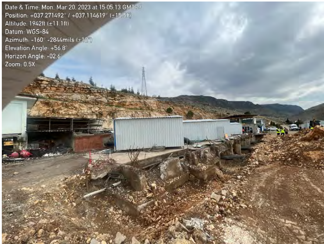
Figure 7.43. Mizmilli pump station (ID No. 79 in Appendix A). Building removed around pumps housed in protective structures.
