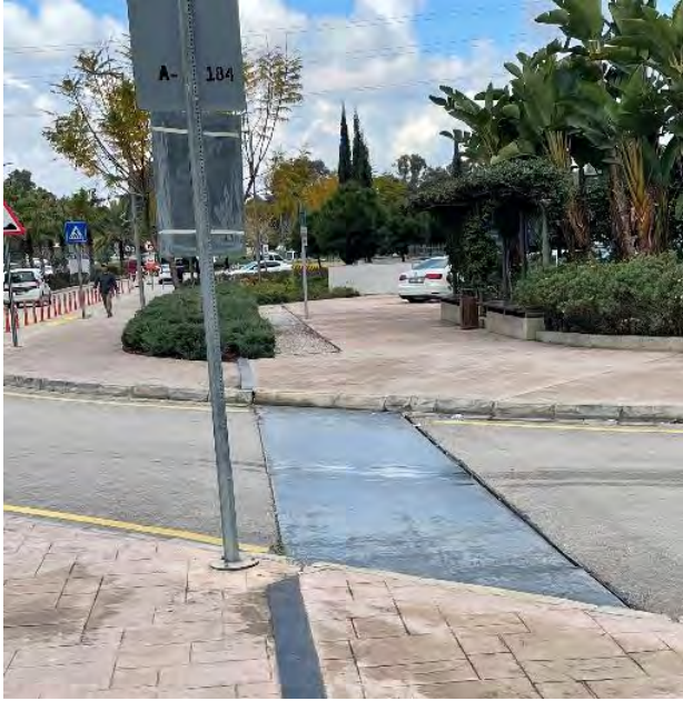
Figure 6.21 Concrete sidewalk crossing the moat gap at Adana City Hospital as observed on March 16, 2023.
