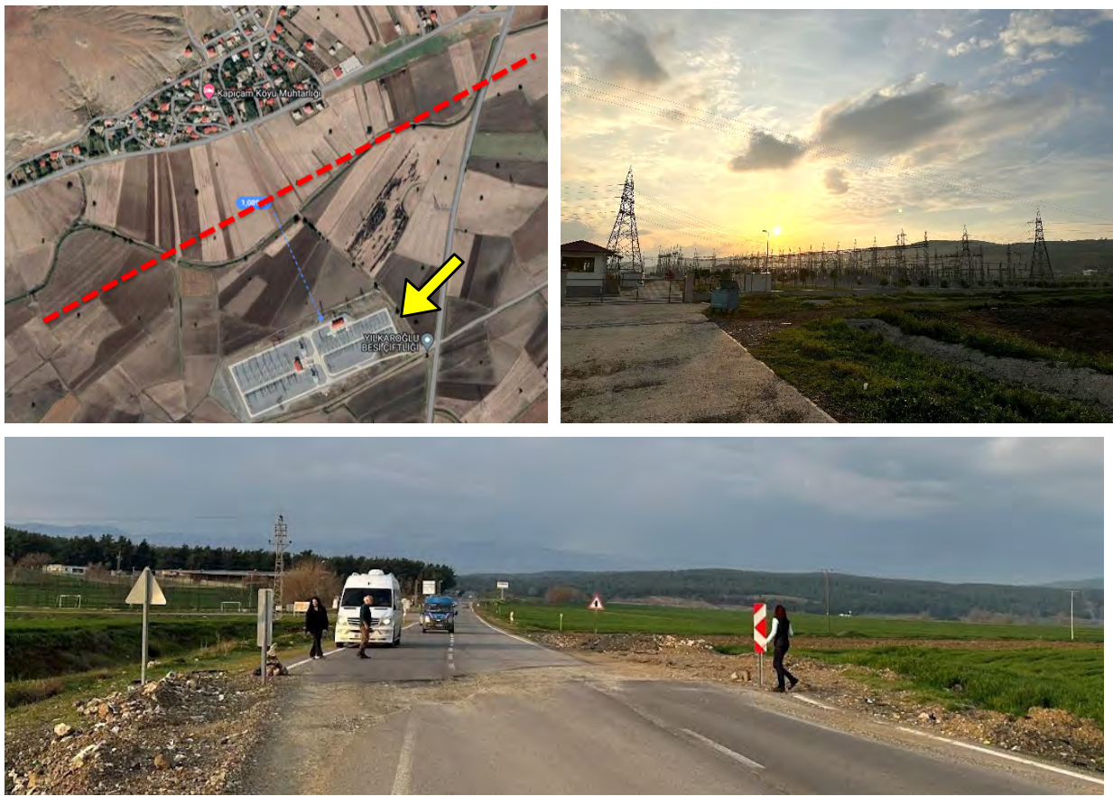
Figure 7.28. Kapiçam substation nearby surface fault rupture (ID No. 165 in Appendix A).
