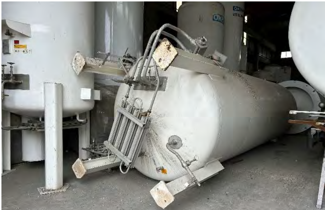
Figure 7.36. Overturned of an unanchored vertical tank at LPG storage facility in Kahramanmaraş (ID 143 in Appendix A).
