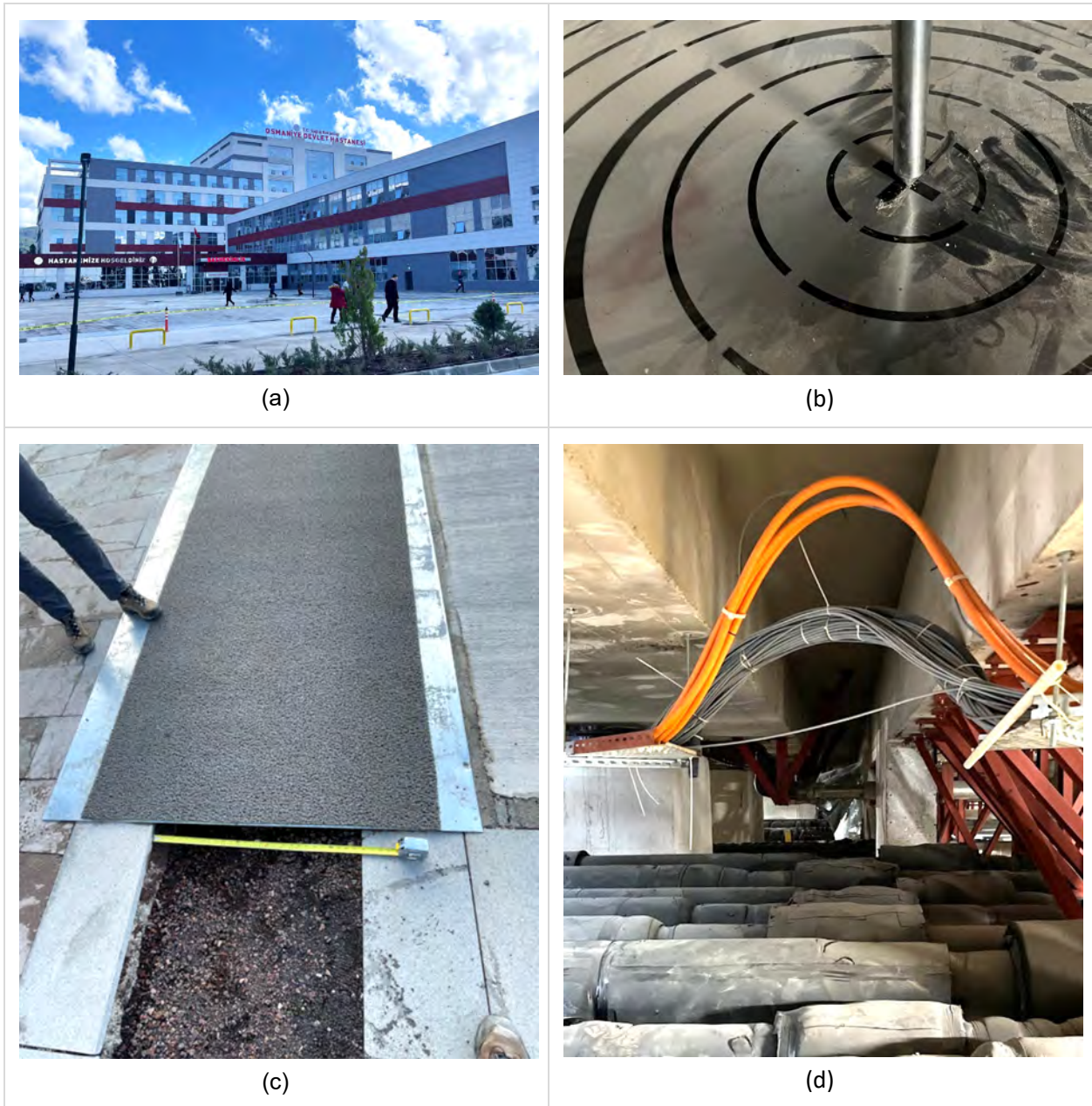
Figure 6.20 Osmaniye Government Hospital as observed on March 16, 2023: (a) building exterior, (b) isolation system scratch plate, (c) moat with soil backfill, (d) Utilities crossing isolation plane.
