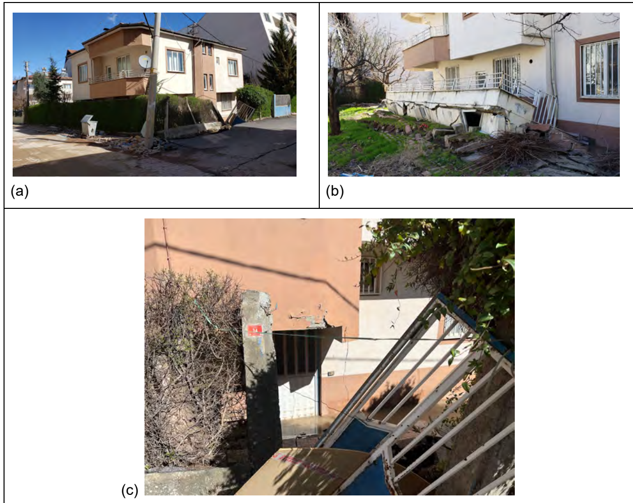
Figure 4.13. Settled two-story residential building with a partial basement in Gölbaşı: (a) view of building from southwest corner (N37.787388°, E37.642918°), (b) collapsed deck over partial basement along north wall (N37.787781°, E37.642868°), (c) front door entrance at southwest corner with over 1.1 m of measured settlement (N37.787494°, E37.643019°). Photographs taken on March 30, 2023.
