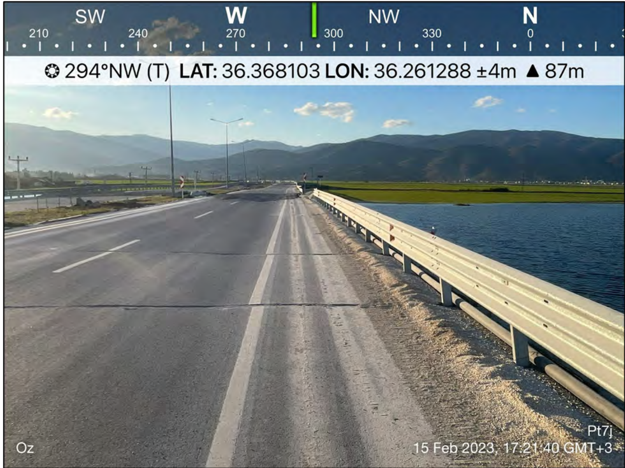
Figure 2.8. February 6, 2023 M7.8 Kahramanmaraş earthquake surface rupture expressed as an approximately 2.1-km-wide deformation zone with secondary fault rupture displacements on the order of centimeters and localized depression. Photo looking along the Hatay Airport access road.
