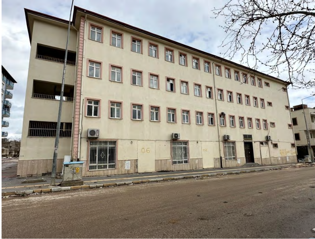
Figure 5.53. Library building in Nurdağı.
