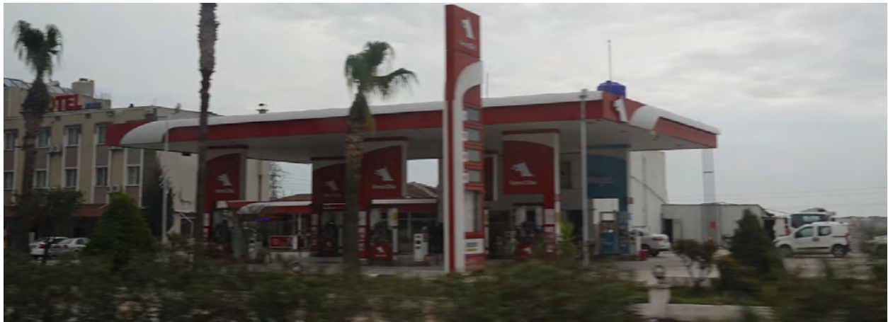
Figure 7.39. Example of petrol station in Antakya without evident structural damage.
