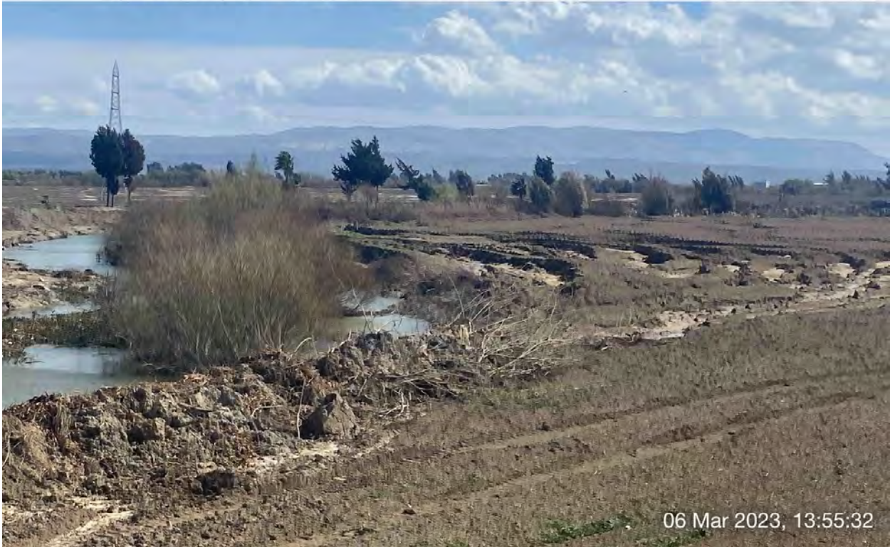
Figure 4.63. Lateral spreading along the Orontes River, south of Demirköprü, Hatay Province.
