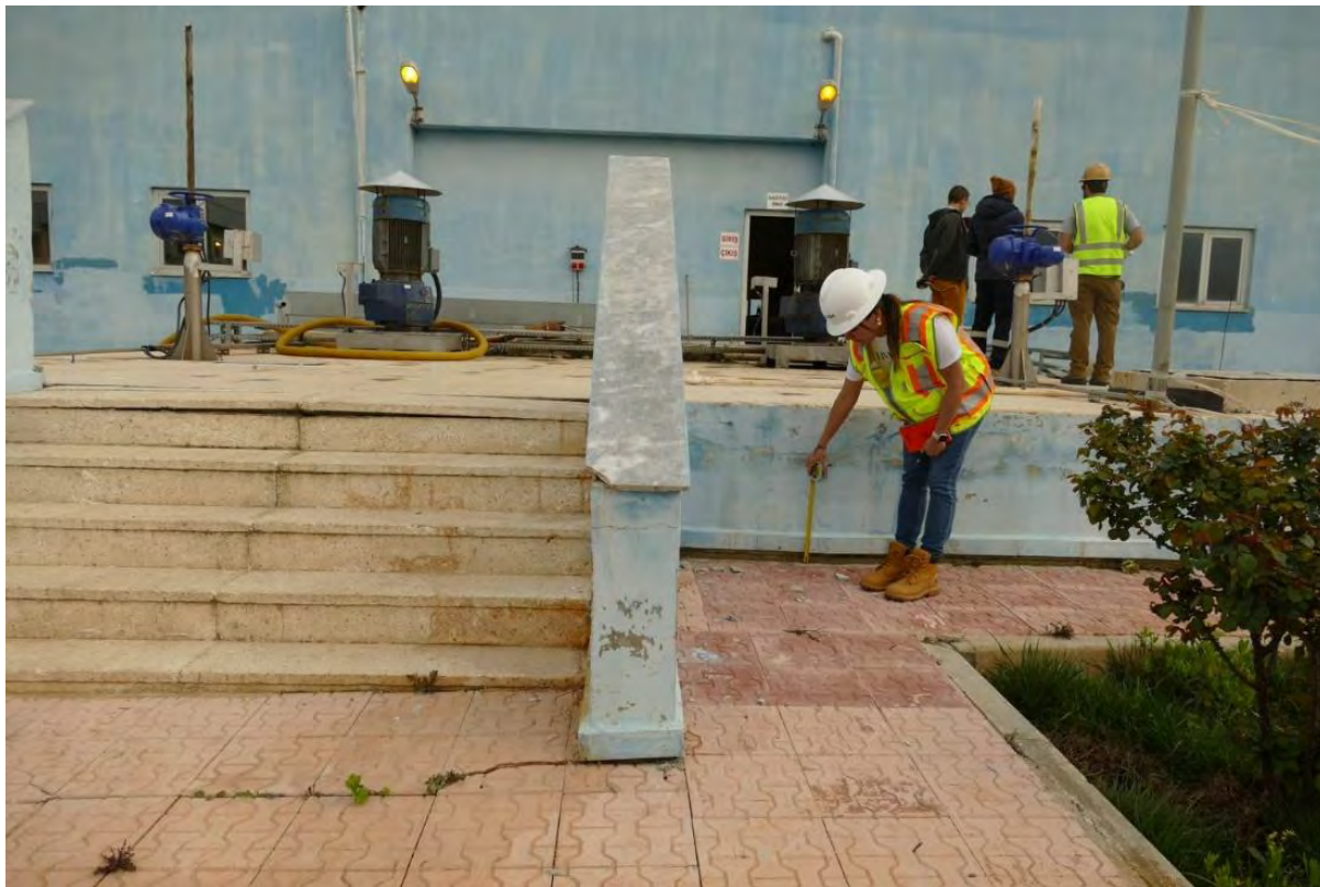
Figure 7.47. Measurement of estimated settlements of approximately 5 cm adjacent to sedimentation process building (background)
