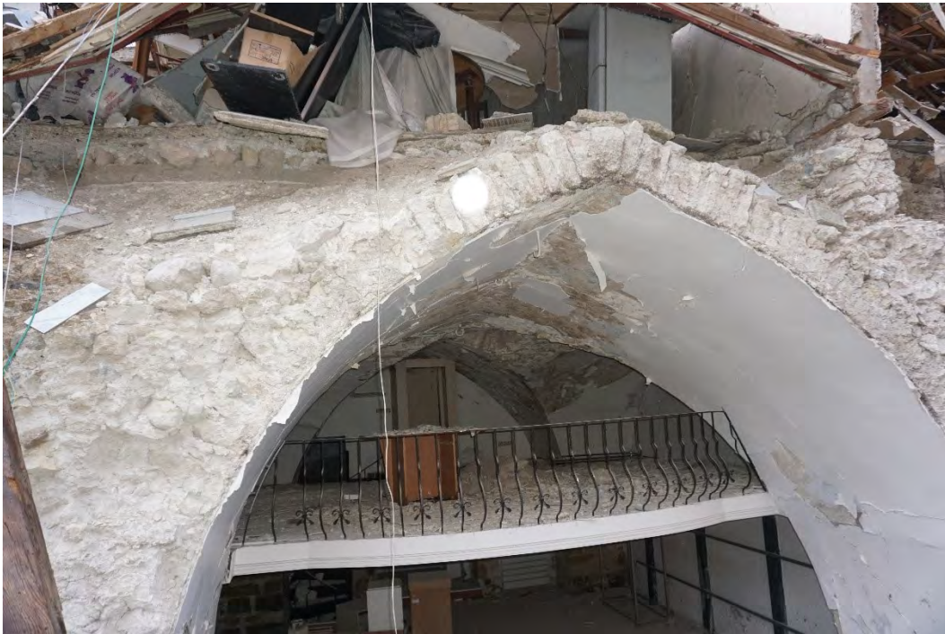
Figure 5.46. Arched structure of the first story.
