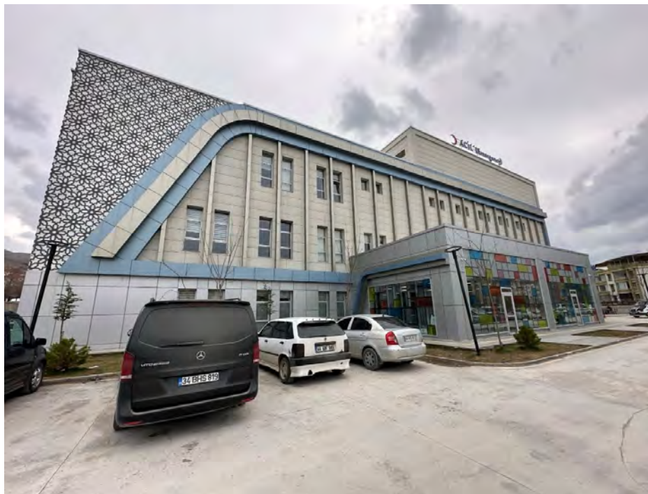
Figure 5.49. Base isolated hospital in service in Malatya.
