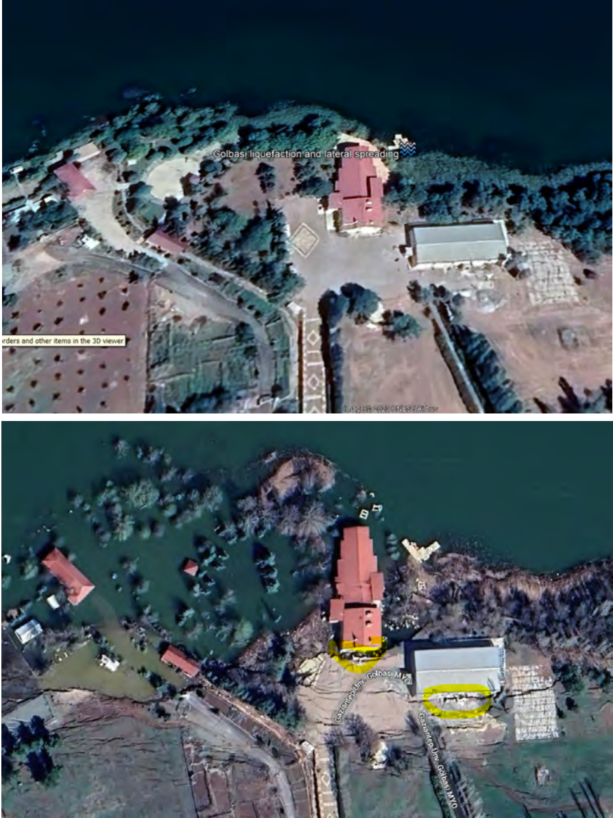
Figure 4.4 Aerial view of the lateral spreading area. Top: Google Earth Image on 9/2022. Bottom: Google Earth image on 3/2023. Referential Coordinates: 37.79° (Lat), 37.65 (Lon)
