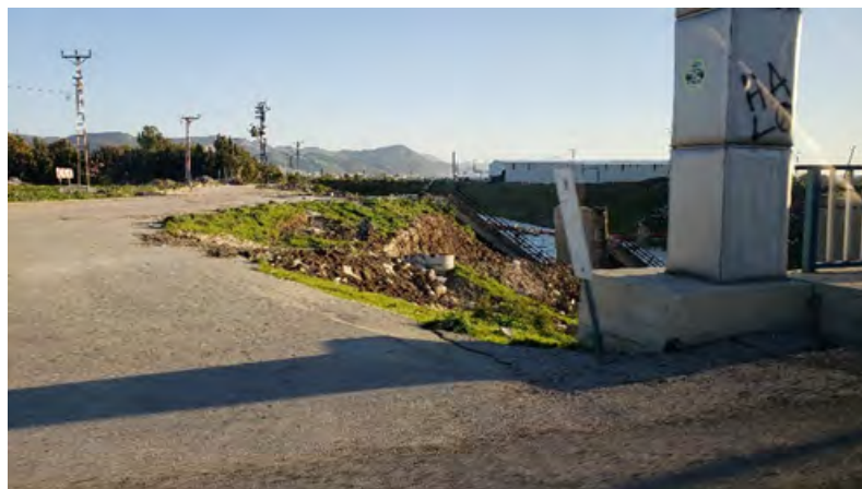
Figure 4.81. Local slumping failure and collapse of old bridge deck along the East bank to the South (background of photo) of the main Hatay Devlet Hospital Bridge (foreground of photo) (N36.27264°, E36.208344°).
