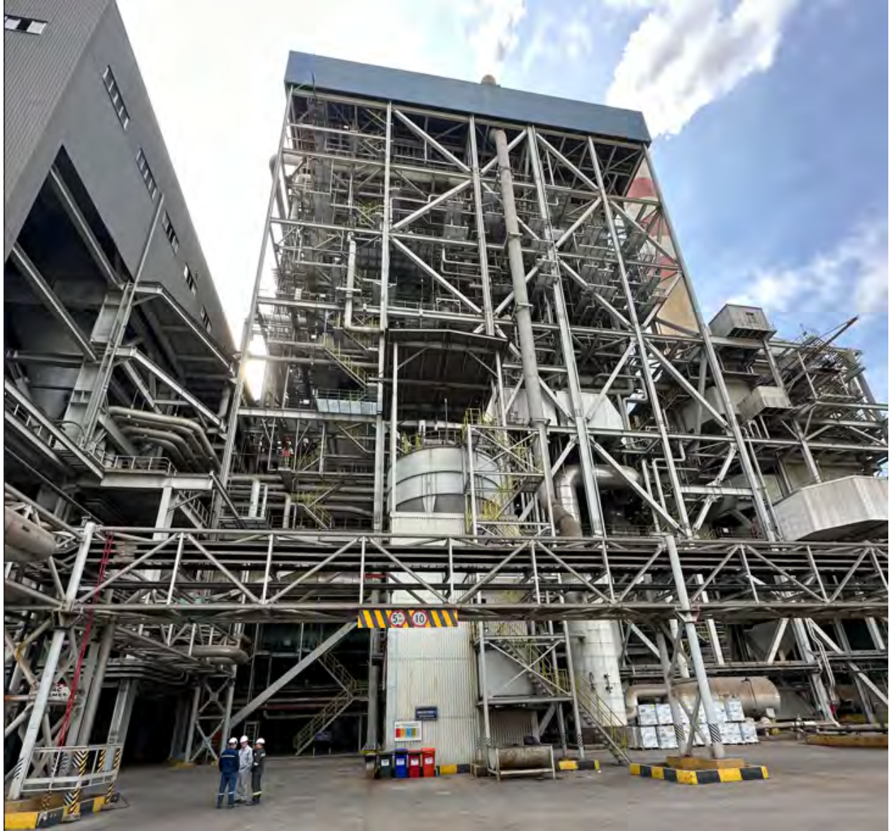
Figure 7.15. Iskenderun plant Unit 2 boiler structure.
