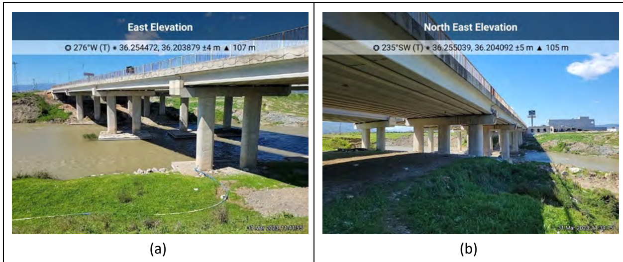
Figure 4.76. Hatay Stadium Bridge crossing the Karasu River from the east end of bridge: (a) east-bound bridge (N36.25472°, E36.203879°), (b) west-bound bridge (N36.255039°, E36.204092°).
