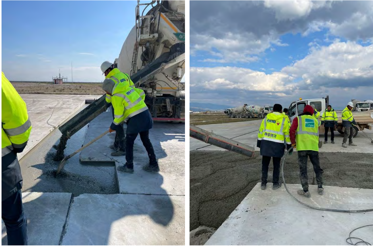
Figure 7.12. Repair work to the Hatay airport runway
