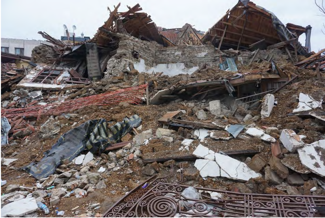
Figure 5.47. Adobe brick masonry debris of a collapsed two-story building.
