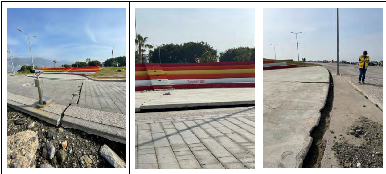
Figure 4.20. Lateral and vertical displacement at the amphitheater located on the waterfront boardwalk. (March 2, 2023; 36.59573N, 36.16206E)
