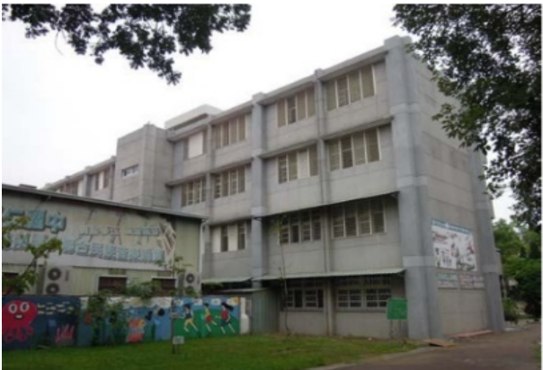
Figure 2.24 Lizhi Building. No structural damage.
