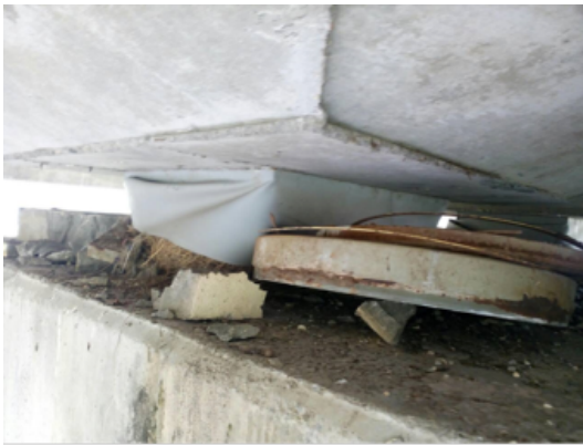
(a) Gaps caused by transverse displacement of 2-way bridges
