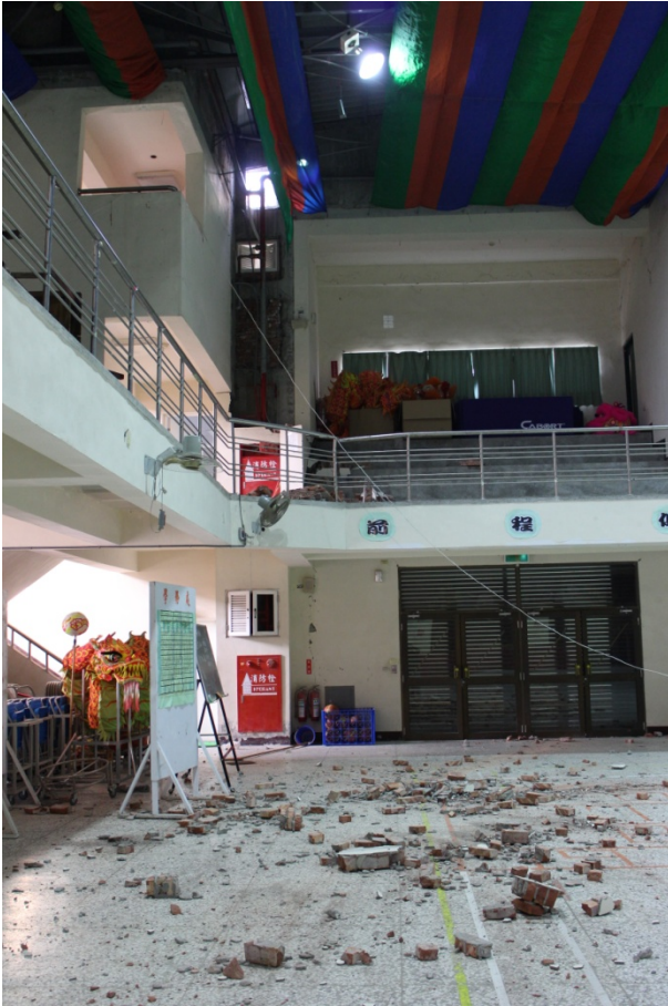
Figure 2.13 Activity Center. Large quantities of red bricks along the pipelines that had fallen off during the earthquake
