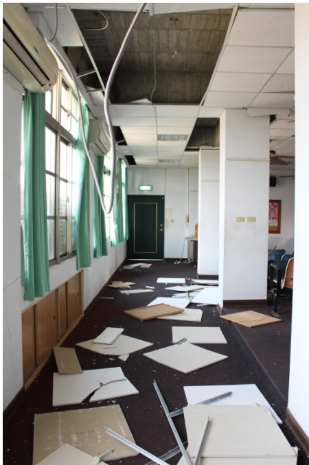
Figure 2.12 Subject Classroom building. Ceiling panels fallen from the light steel frame
