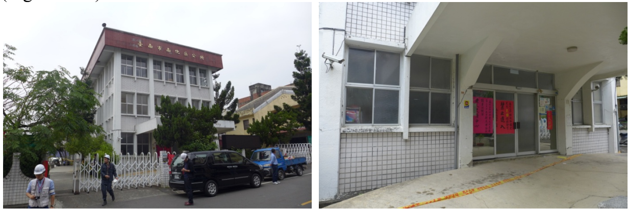
Figure 2.29 Nanhua District Office, a 3-story reinforced concrete building.
