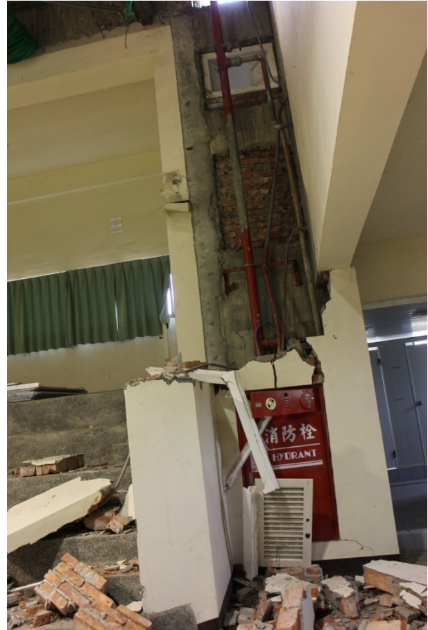
Figure 2.13 Activity Center. Large quantities of red bricks along the pipelines that had fallen off during the earthquake
