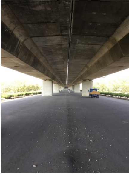
(a) Gaps caused by transverse displacement of 2-way bridges
