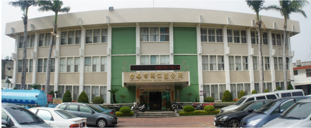
Figure 2.31 Gueiren District Office, a 3-story reinforced concrete building
