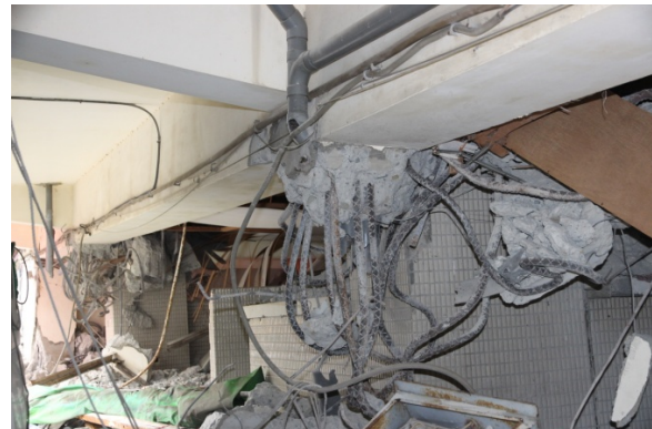
(b) Axial damage of the columns
