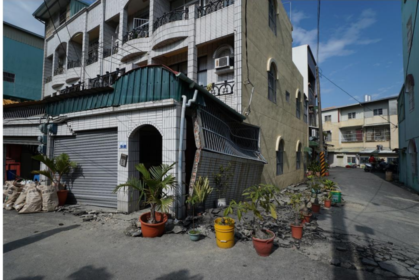
(A) Sinking and tipping of buildings
