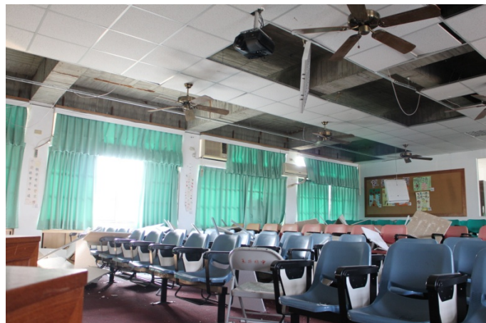
Figure 2.12 Subject Classroom building. Ceiling panels fallen from the light steel frame
