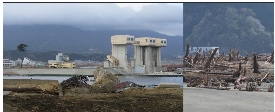
Figure 6. Left: the sole surviving pine tree out of a forest of 70,000 trees planted to protect the Rikuzentakata coast from tsunamis and storm surge. The towers on the left are part of the tsunami gates built to prevent tsunami surges from flooding the Kesen River. Right: the remains of the pine forest. Mature pine tree trunks were 20-40 cm in diameter and typically snapped 1-2 m above the ground (photos: L. Dengler).
