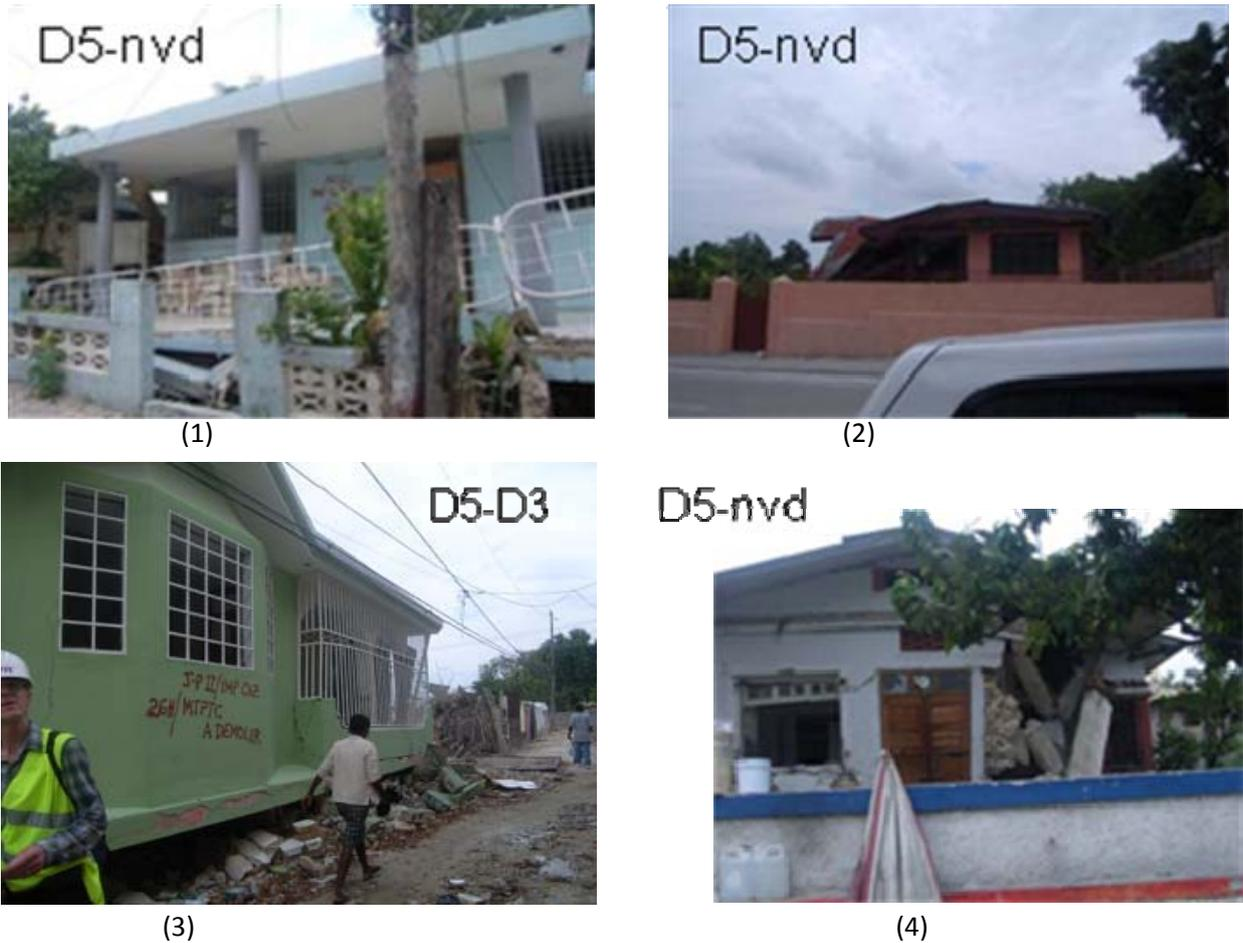
Figure 10. Examples of D5 (EEFIT) – nvd or D3 in Pictometry
