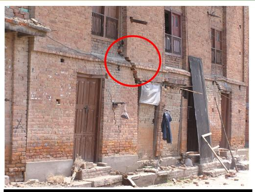
Severe damage to the walls due to the absence of lintel band around openings
