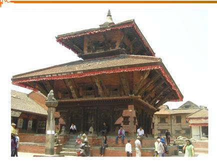
Most of the temples were built in pagoda style, having timber frames and brick masonry walls. The walls were of random rubble masonry core and dressed with brick masonry.
