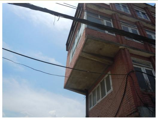
Due to the extension of masonry wall beyond column line, the columns supporting the projection will be overstressed and the outer wall will also susceptible to damage due to lesser stiffness.
