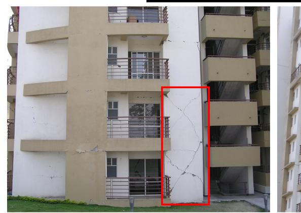
Diagonal cracks in the infill walls of high-rise buildings Combined in-plane and out-of-plane failure of infill wall
