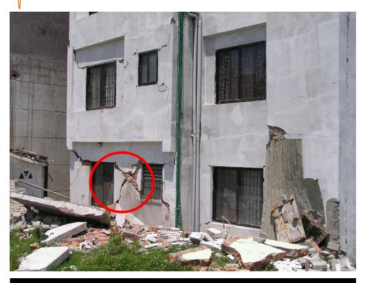
Diagonal cracks in the wall due to lack of confining RC band around openings
