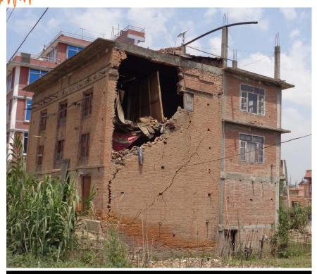
Out-of-plane failure of the wall and step-type diagonal cracks
